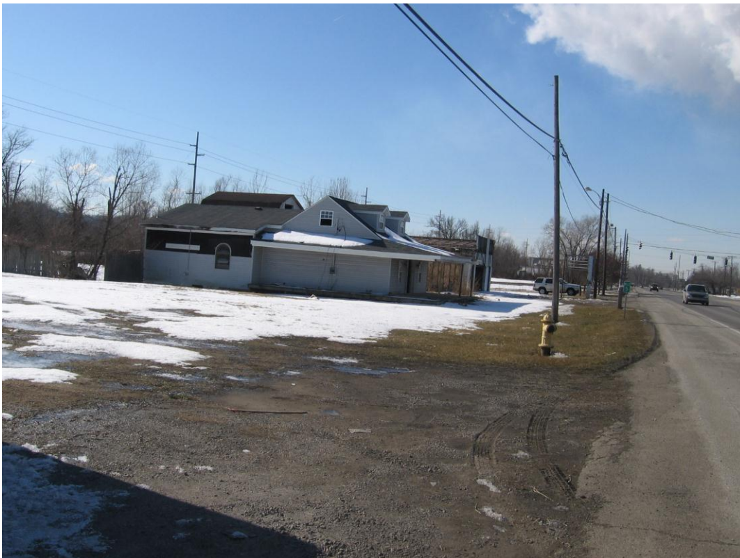
Looking south from northern perimeter toward the existing structures
