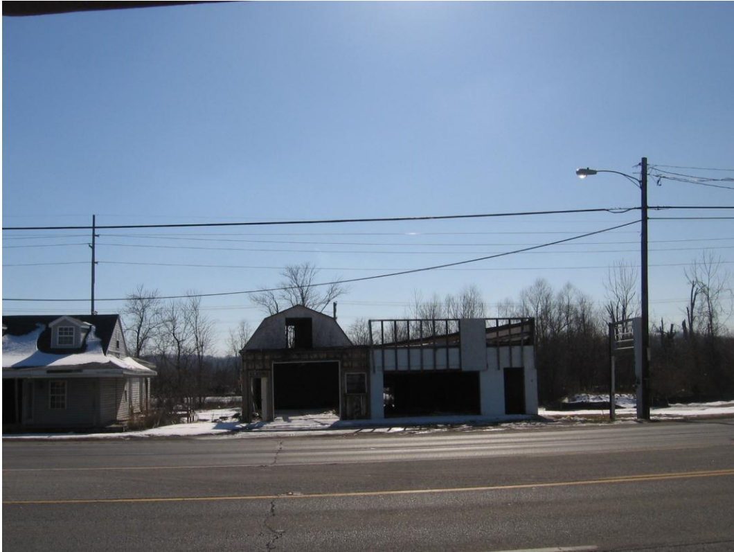
Southern portion of the site
