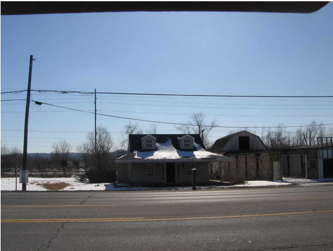
Middle portion of the site
