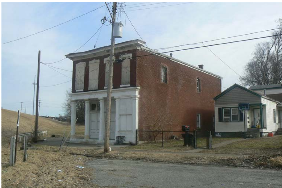
Side View – 3200 Rudd Avenue
