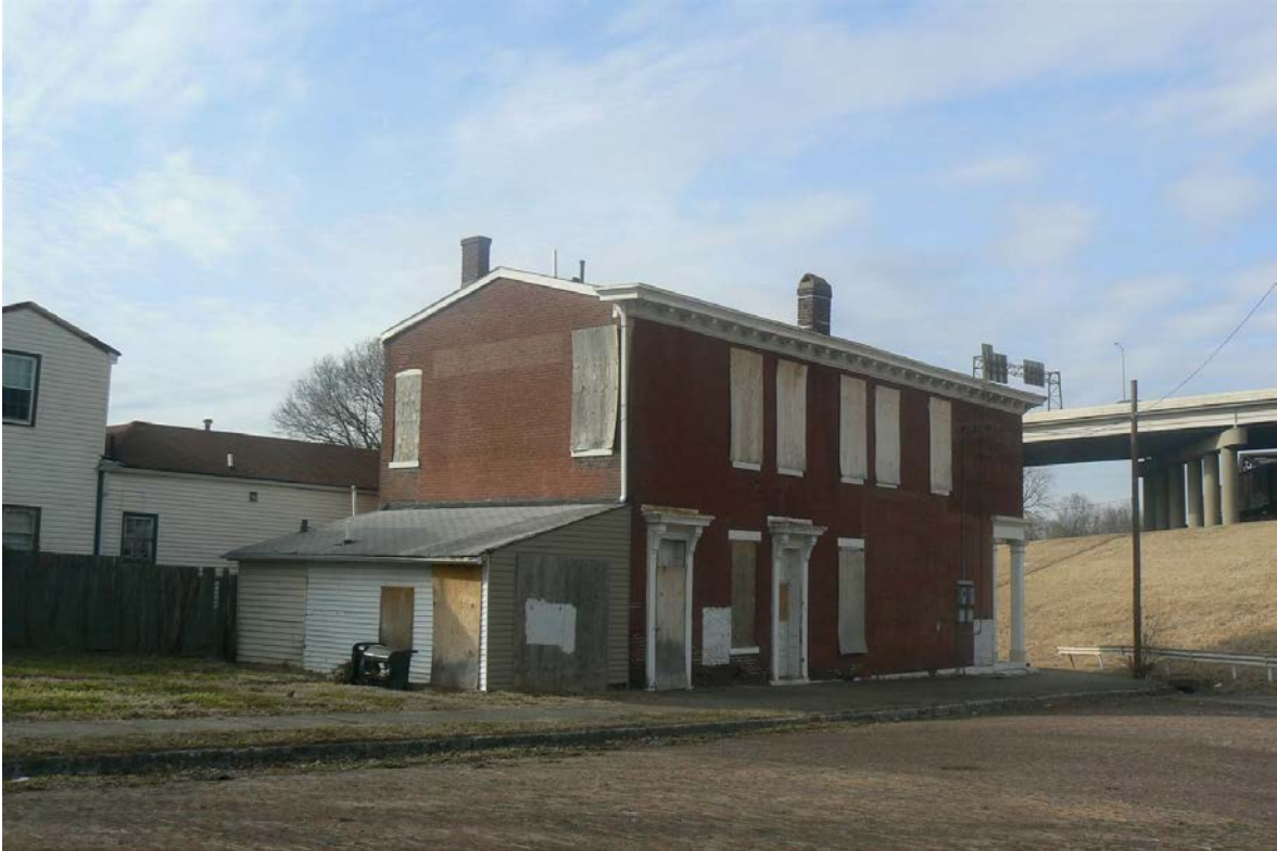
Side View – 3200 Rudd Avenue
