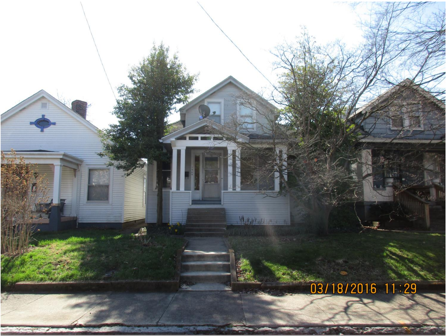
The front of 1904 Stevens Ave. (looking south).
