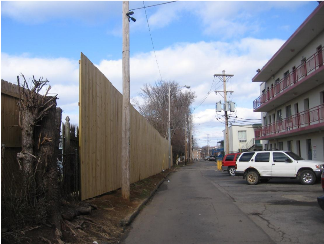
Portion of the new fencing which is 12 feet tall along the rear of the property
