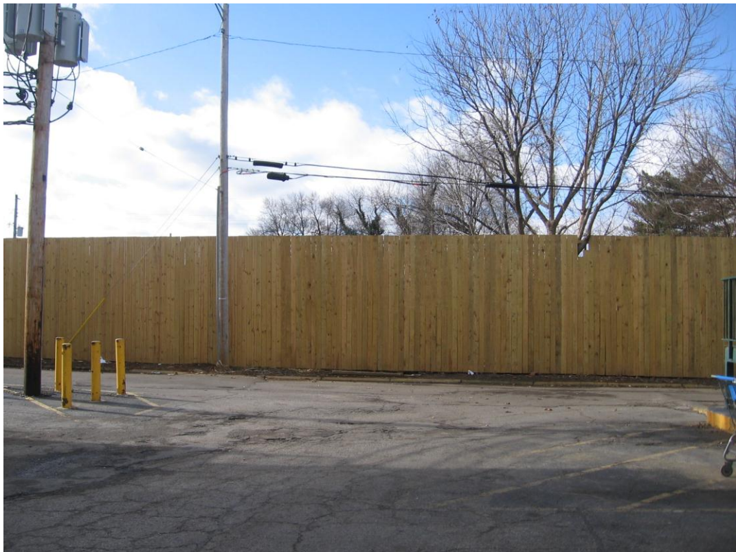
12 feet fencing along rear of property
