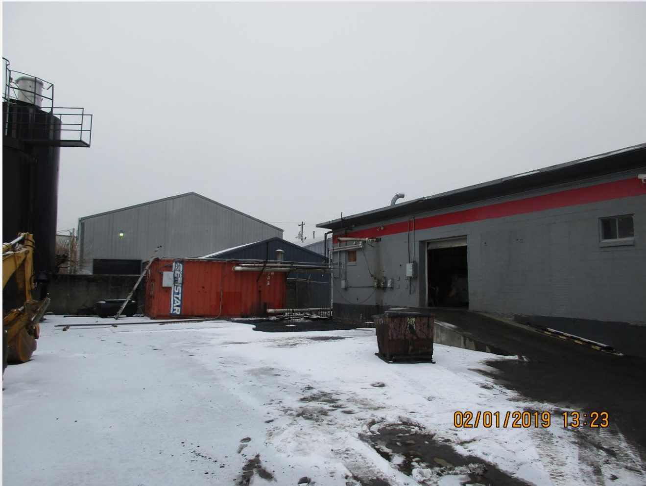
Silo site looking south.
