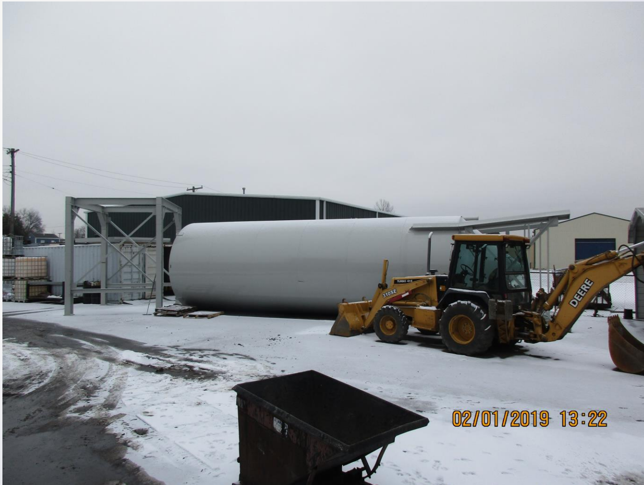
Silo and base.
