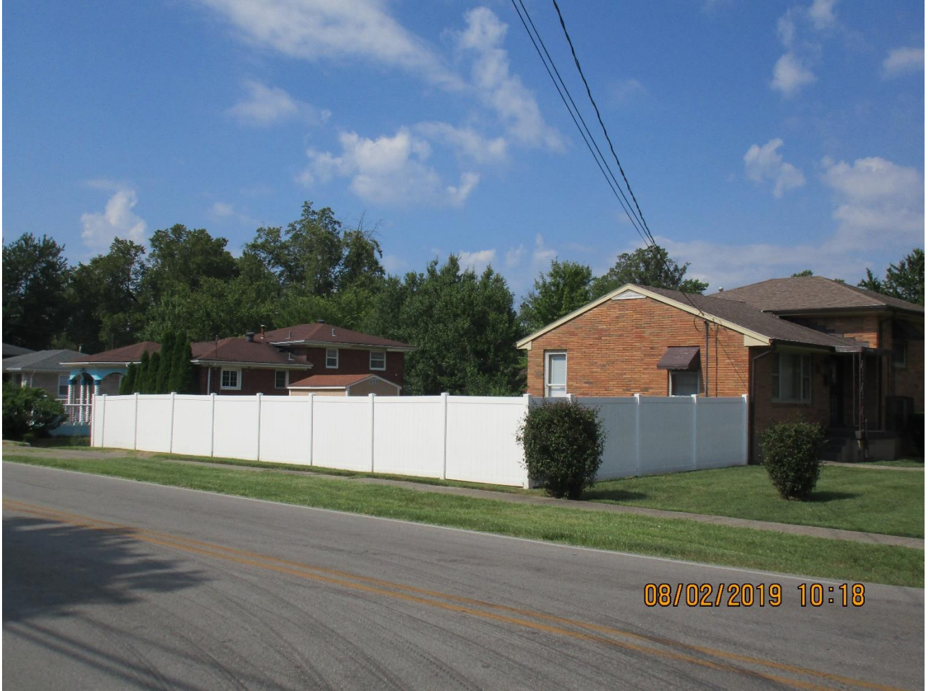
Fence from Jeanine Drive (street side yard).
