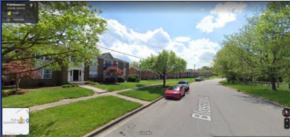
Apartments along Blossom Lane
