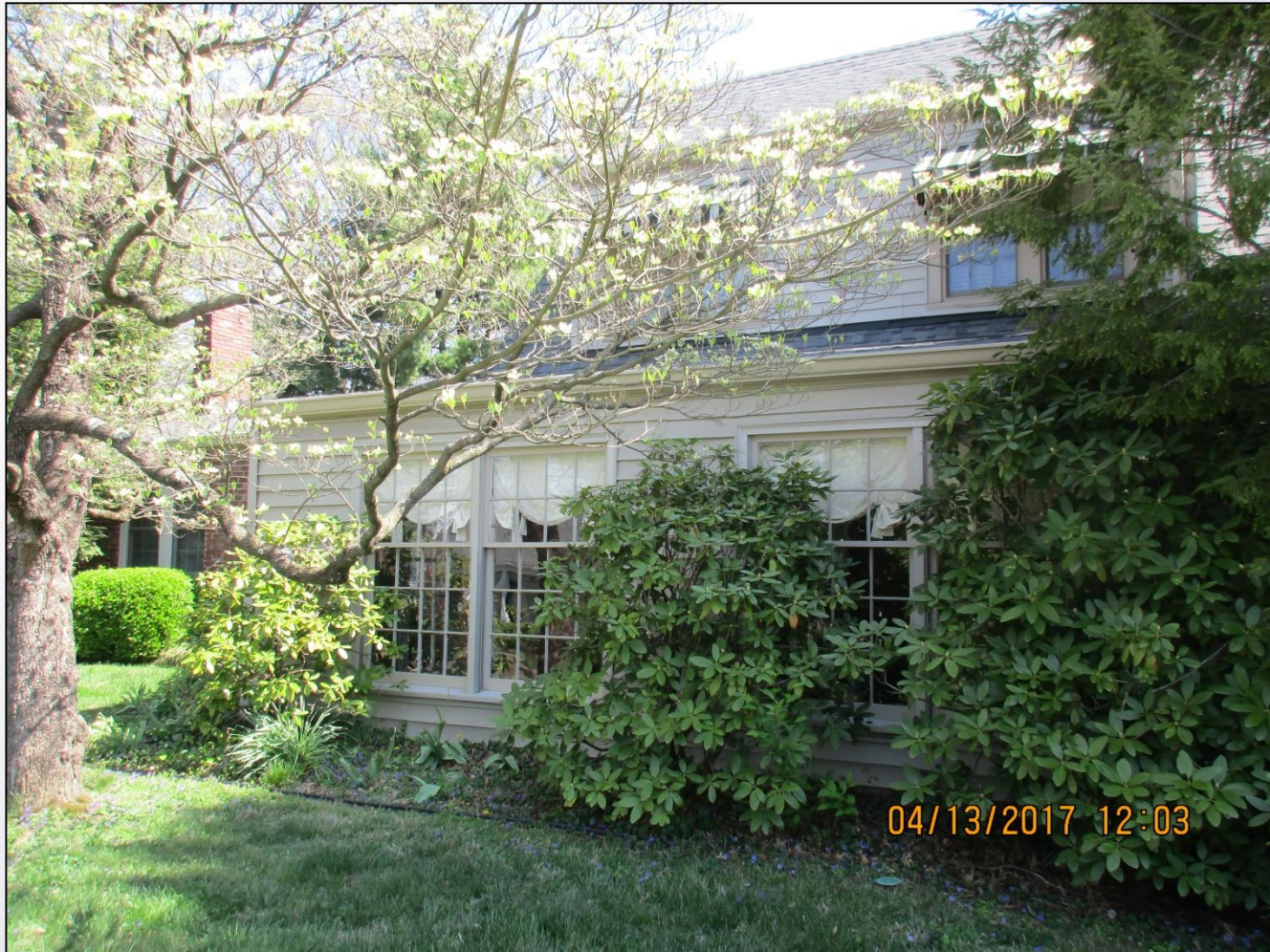
The existing sun porch.
