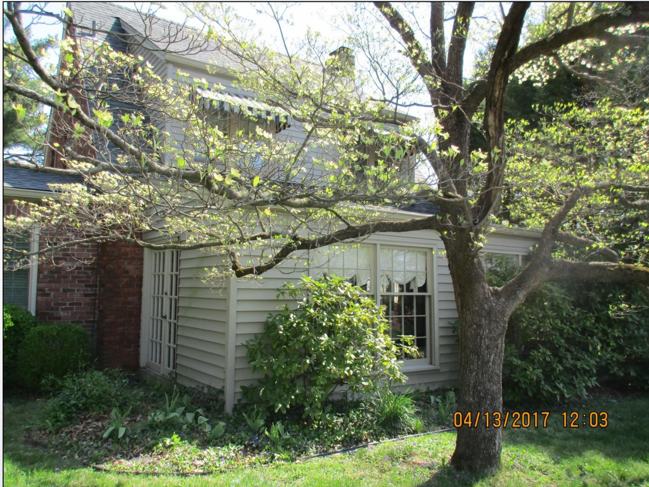
The existing sun porch.
