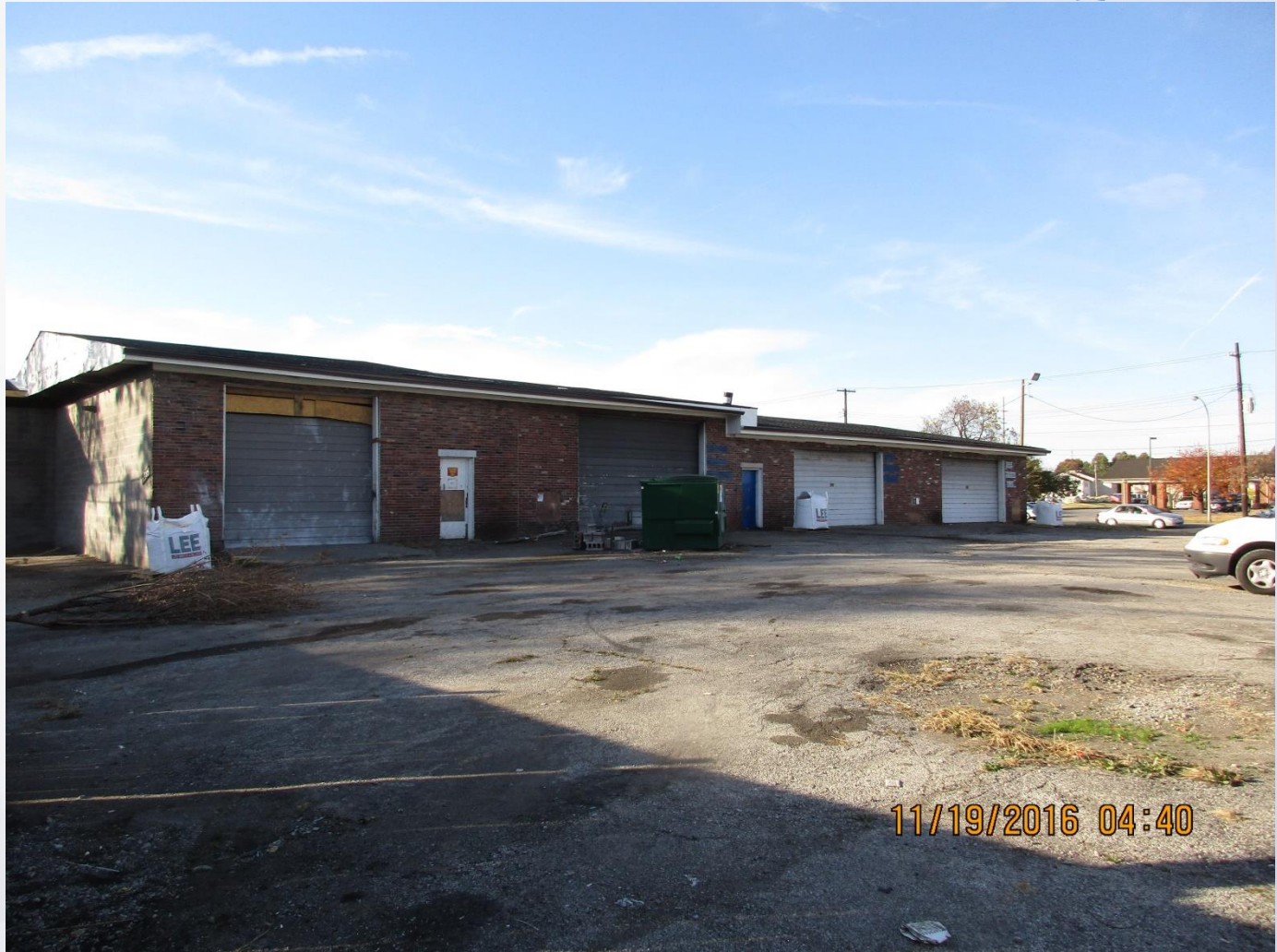
The existing building, looking Northwest towards Broadway.
