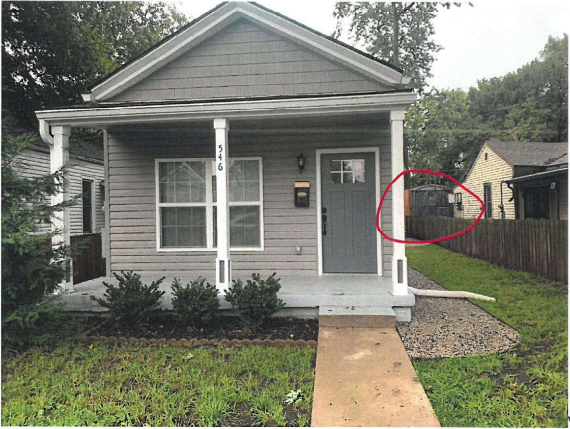
Photo 4 (Front Wainwright Avenue view): my fence is barely visible from the front of the property and does not affect street aesthetics. In fact, Mr. Rice's fence is much more visible.
