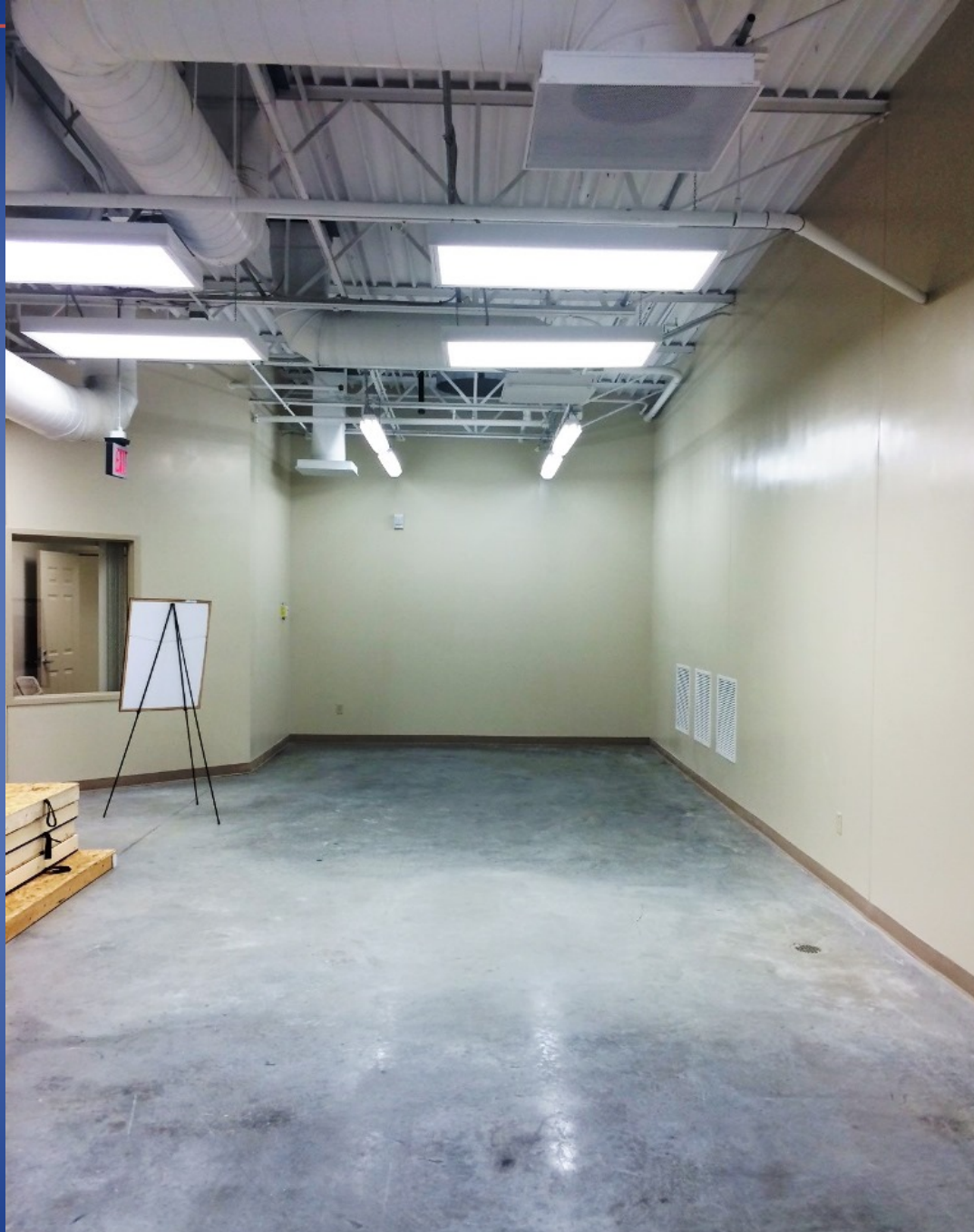
Proposed crematory room; note viewing window to left of photograph
