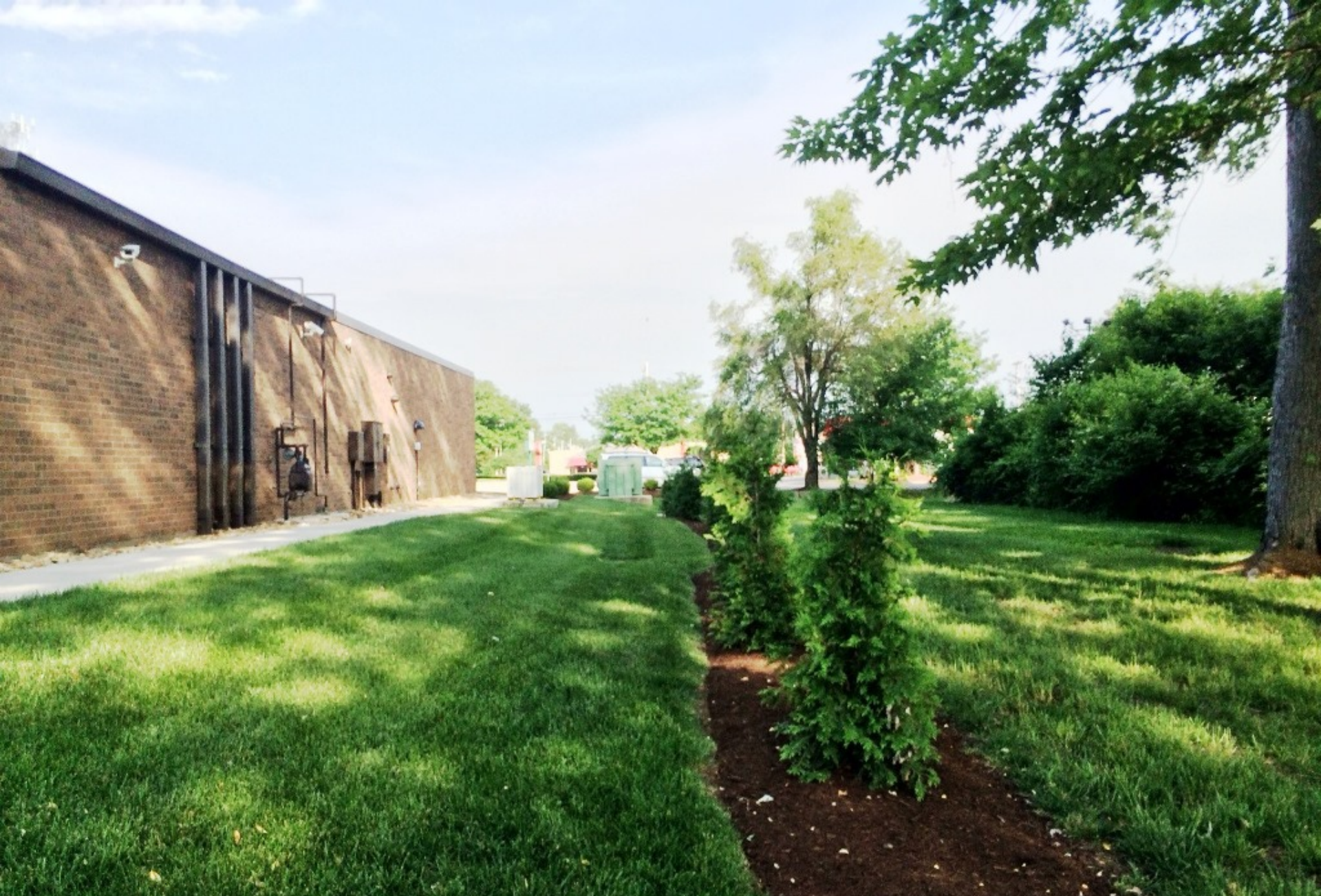
East view of south side of Newcomer Funeral Home building; to right of photograph is the existing drainage swale and new landscaping along south property line
