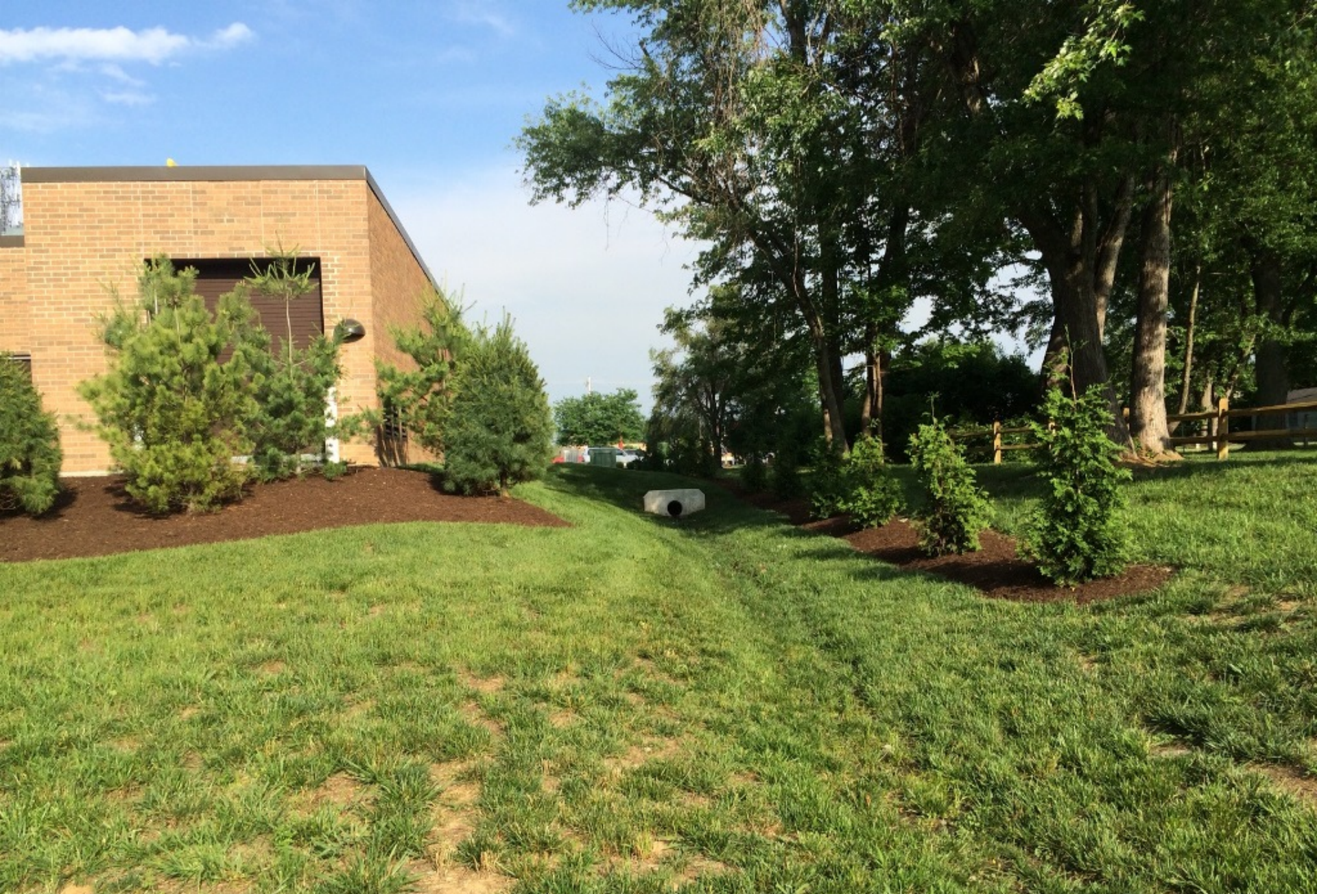
East view of rear of Newcomer Funeral Home building; to right of photograph is the existing drainage swale and new landscaping along south property line
