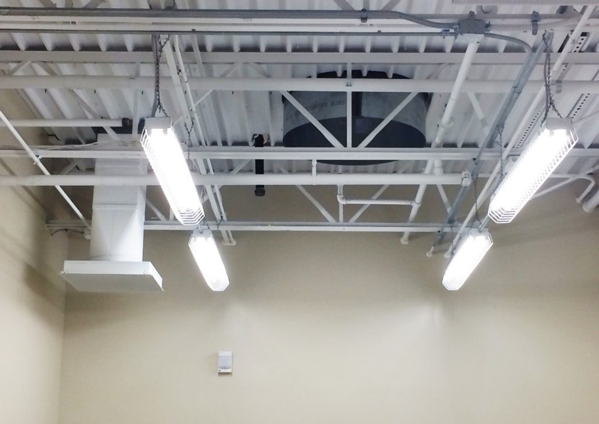
Proposed crematory room ventilation ductwork
