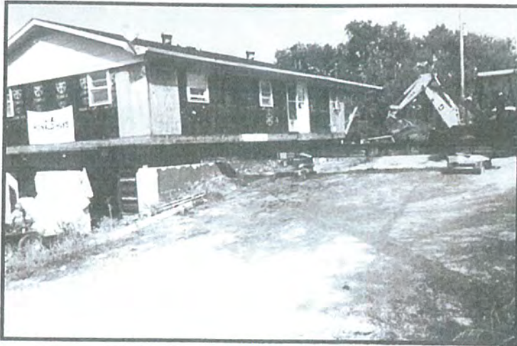
Installing 12" slide beams. Using 6" uphill grade.
