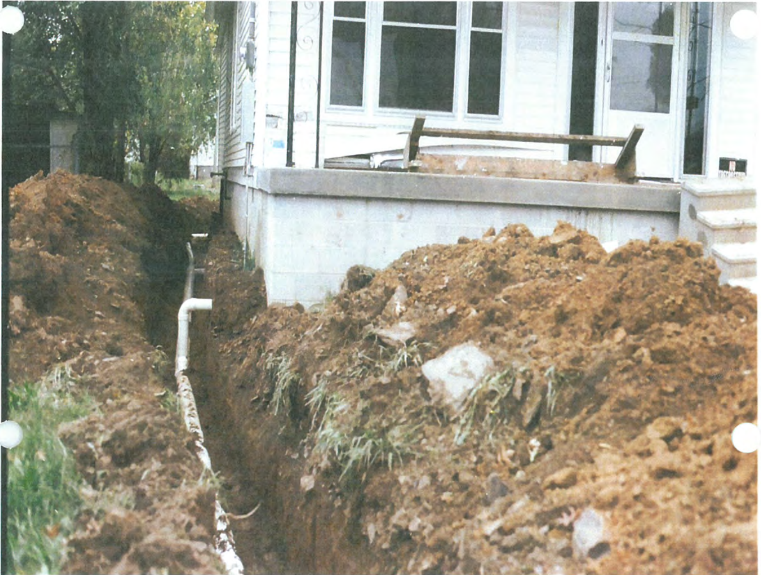
1996 - Installing storm drain plumbing after house move.
