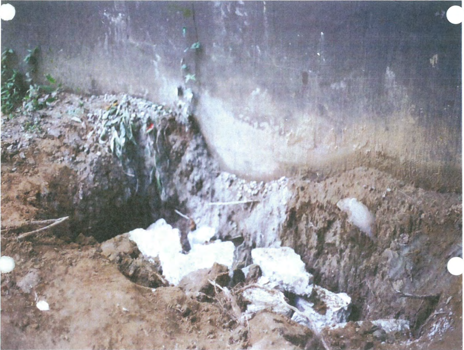
1999 - Foundation repair job.
