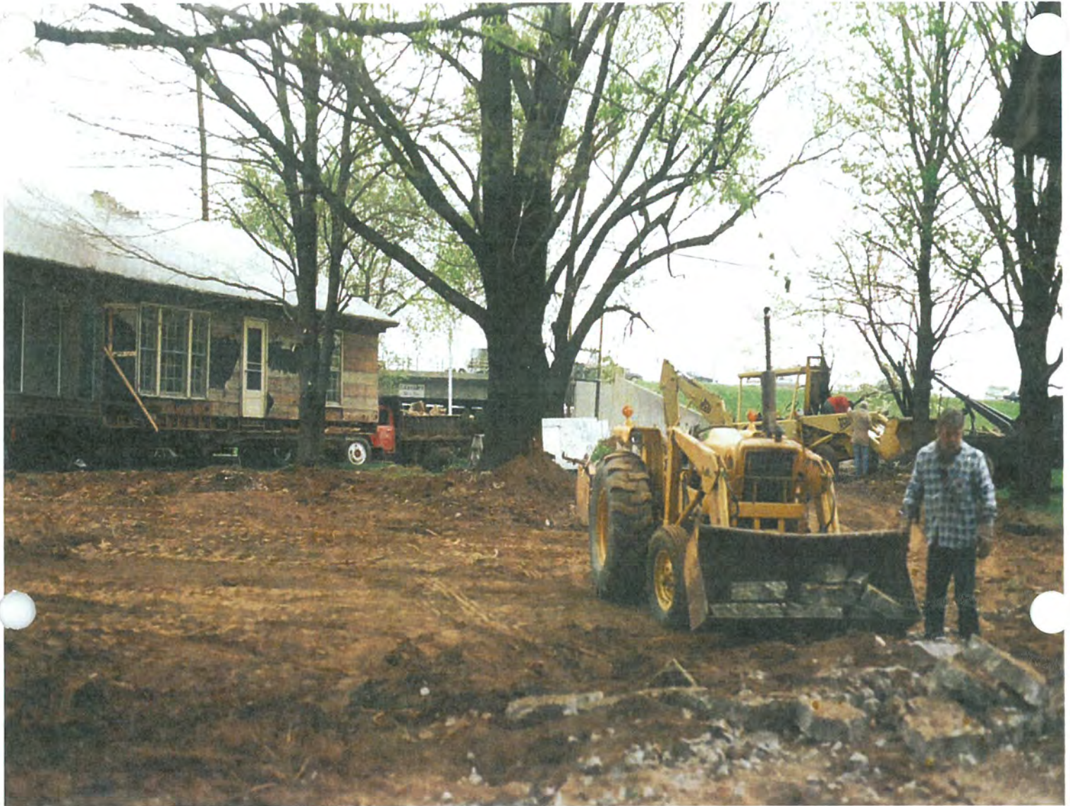
1997 - House moving job, clearing and cleaning lot.
