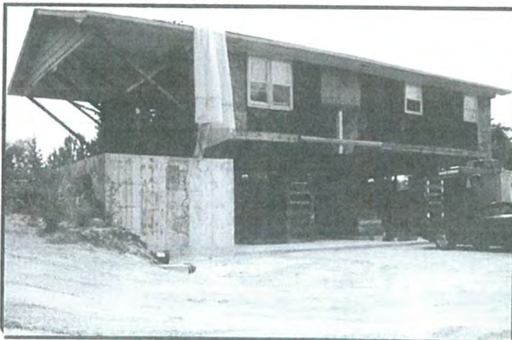
Squared over foundation and ready to be lowered onto foundation.
