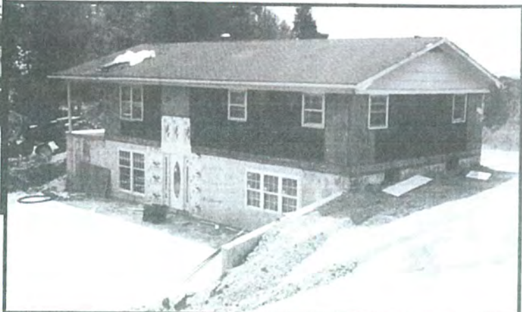
Finished and ready for siding.
