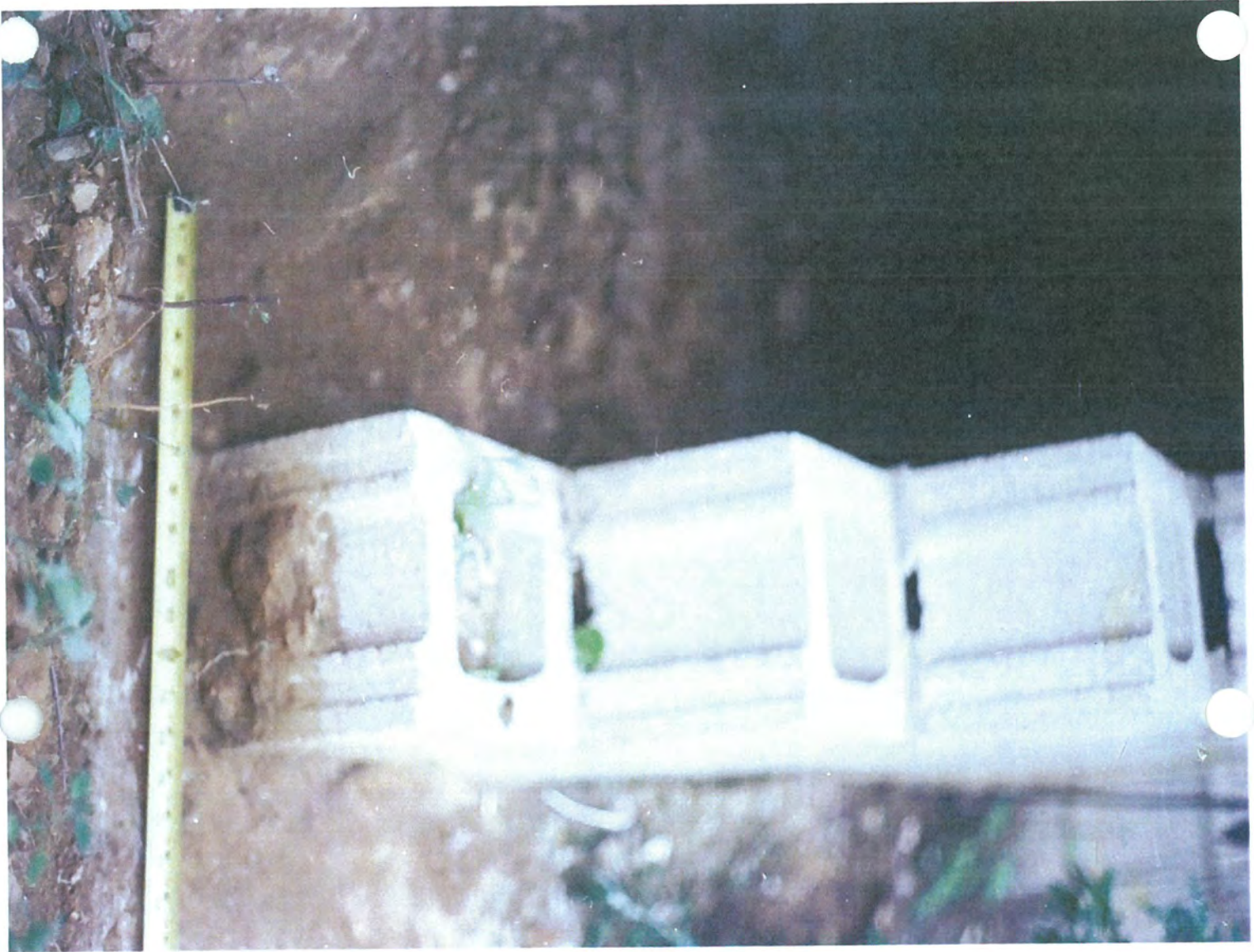
1993 - Mac Sawyers House and Building movers adding supports to sagging foundation.
