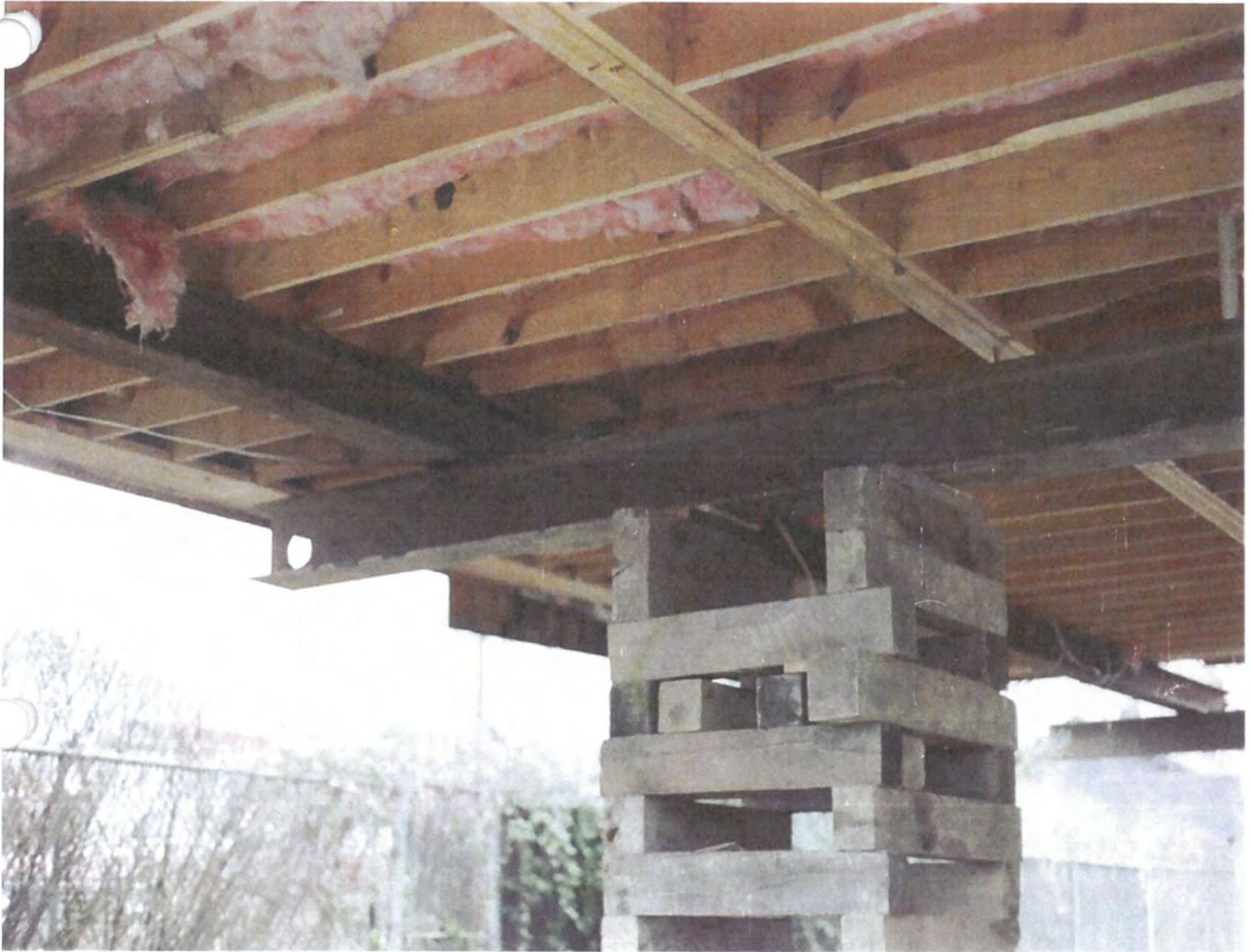
1998 - Steel beams under house at house moving job.
