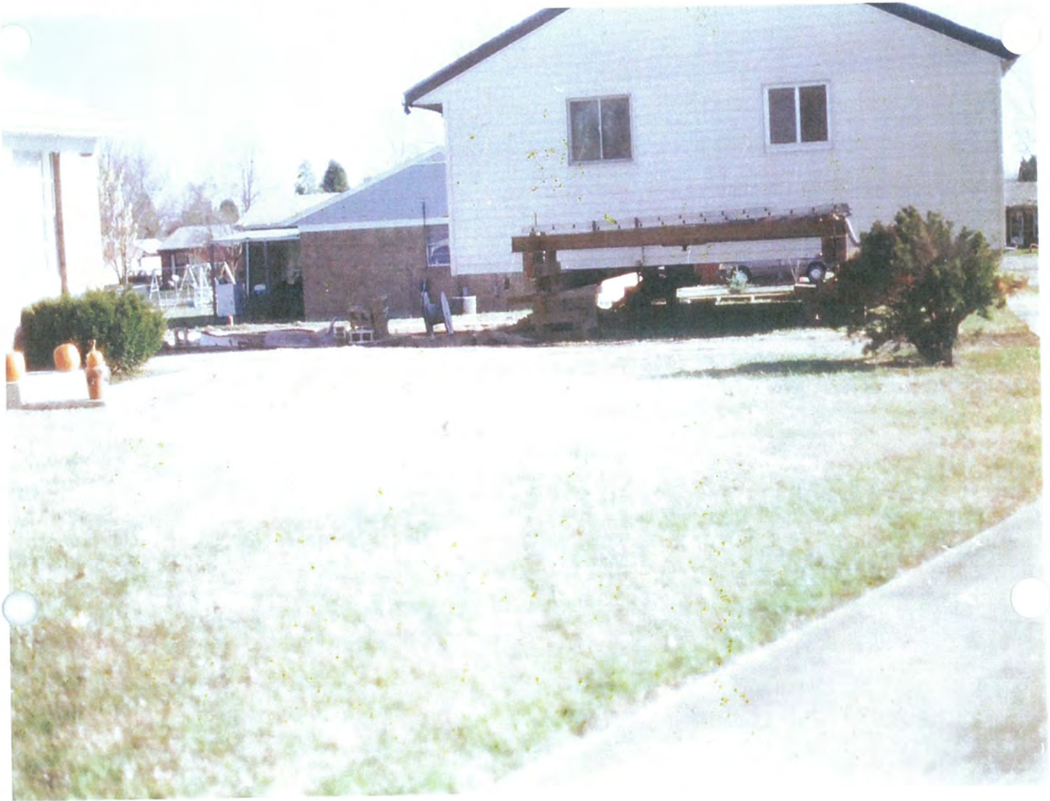
1992 - House moving job, house ready to head to new home.
