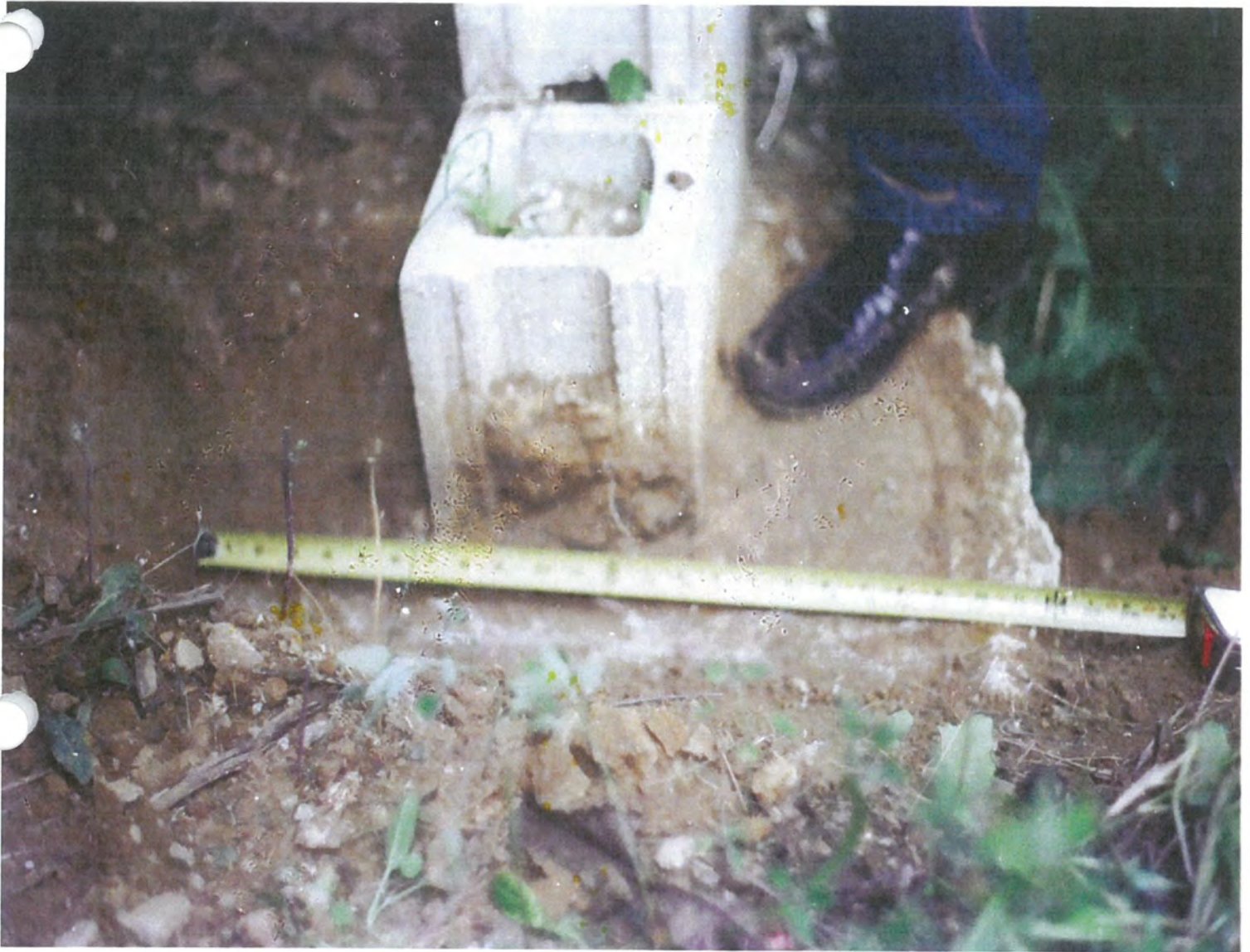
1993 - Mac Sawyers House and Building movers adding supports to sagging foundation.
