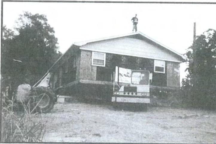
Hard move around pole and foundation - only 6" clearance. Used Terminal Tractor with hydraulic jacking fifth wheel.
