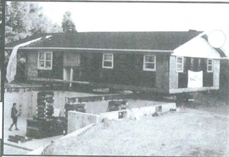
Sliding onto new foundation using Hevi-Haul skates!
