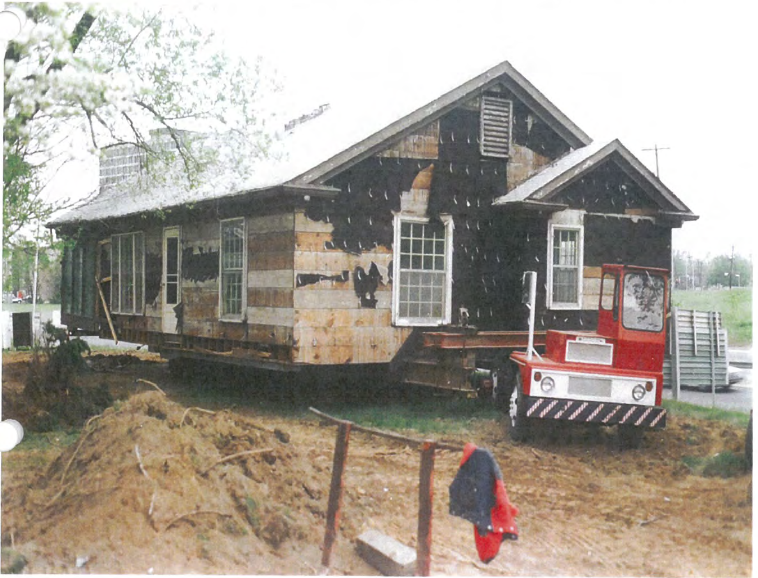
1997 - Mac Sawyers House and Building Movers moving a house.
