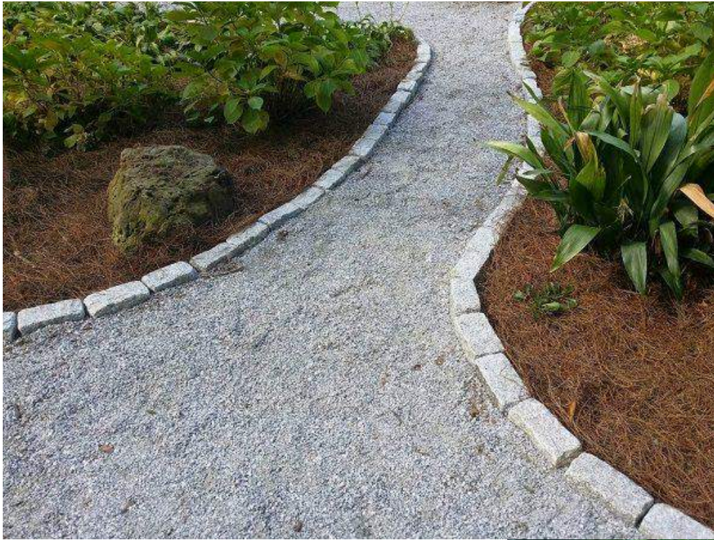
PAVER-EDGED GRAVEL PATH
