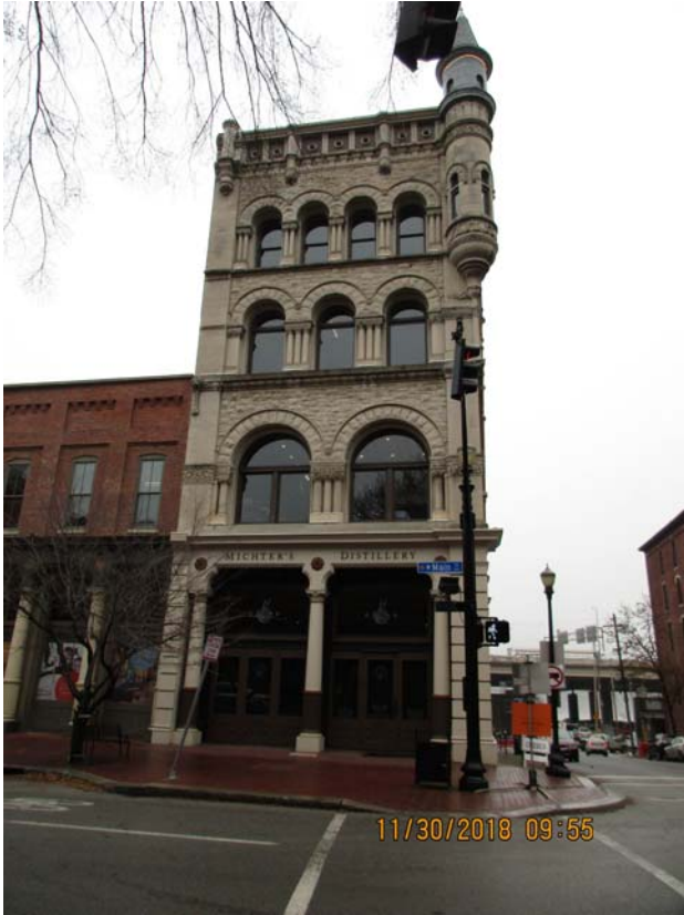
Front of building from Main Street
