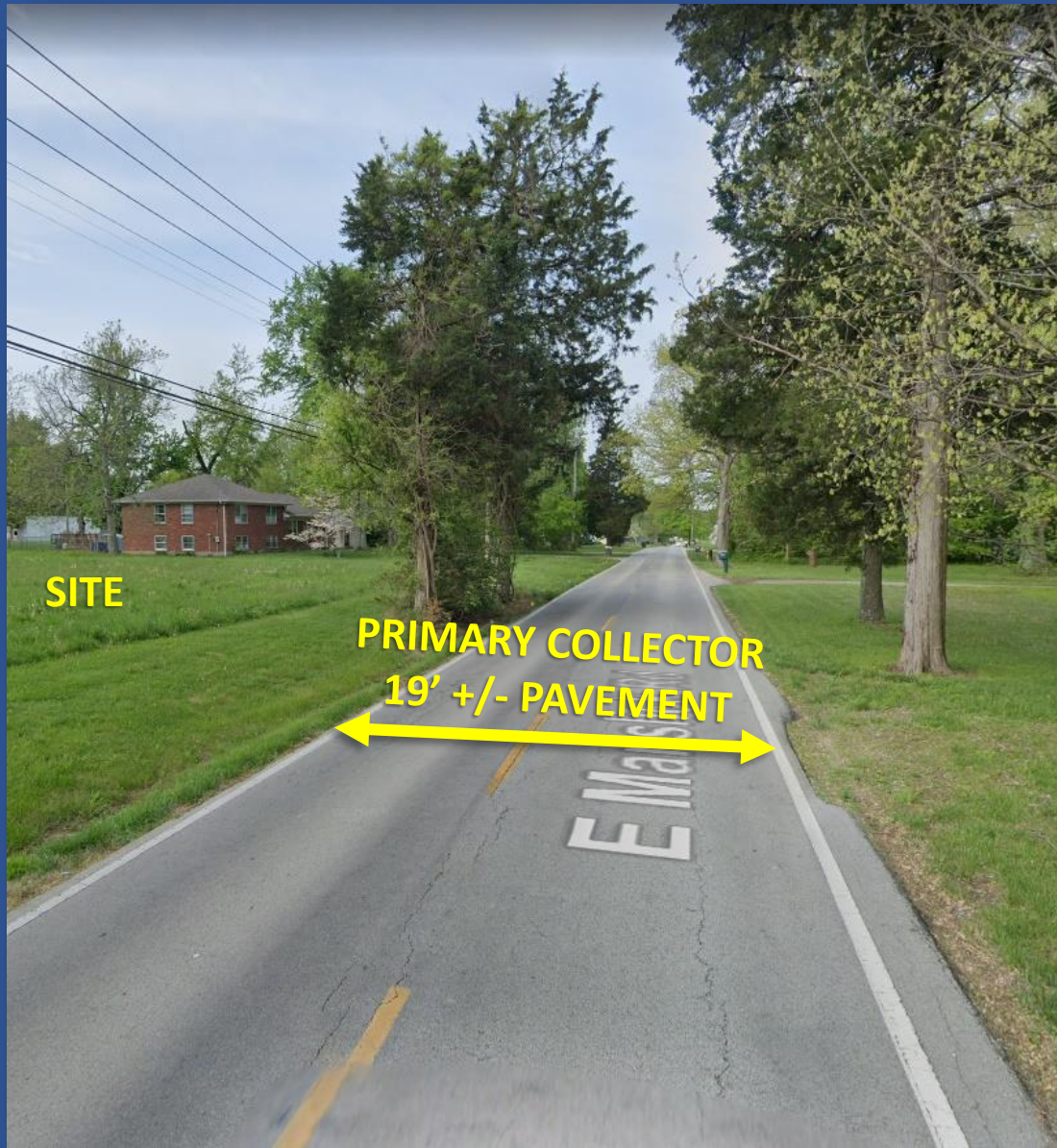
E. MANSCLICK RD LOOKING WEST
