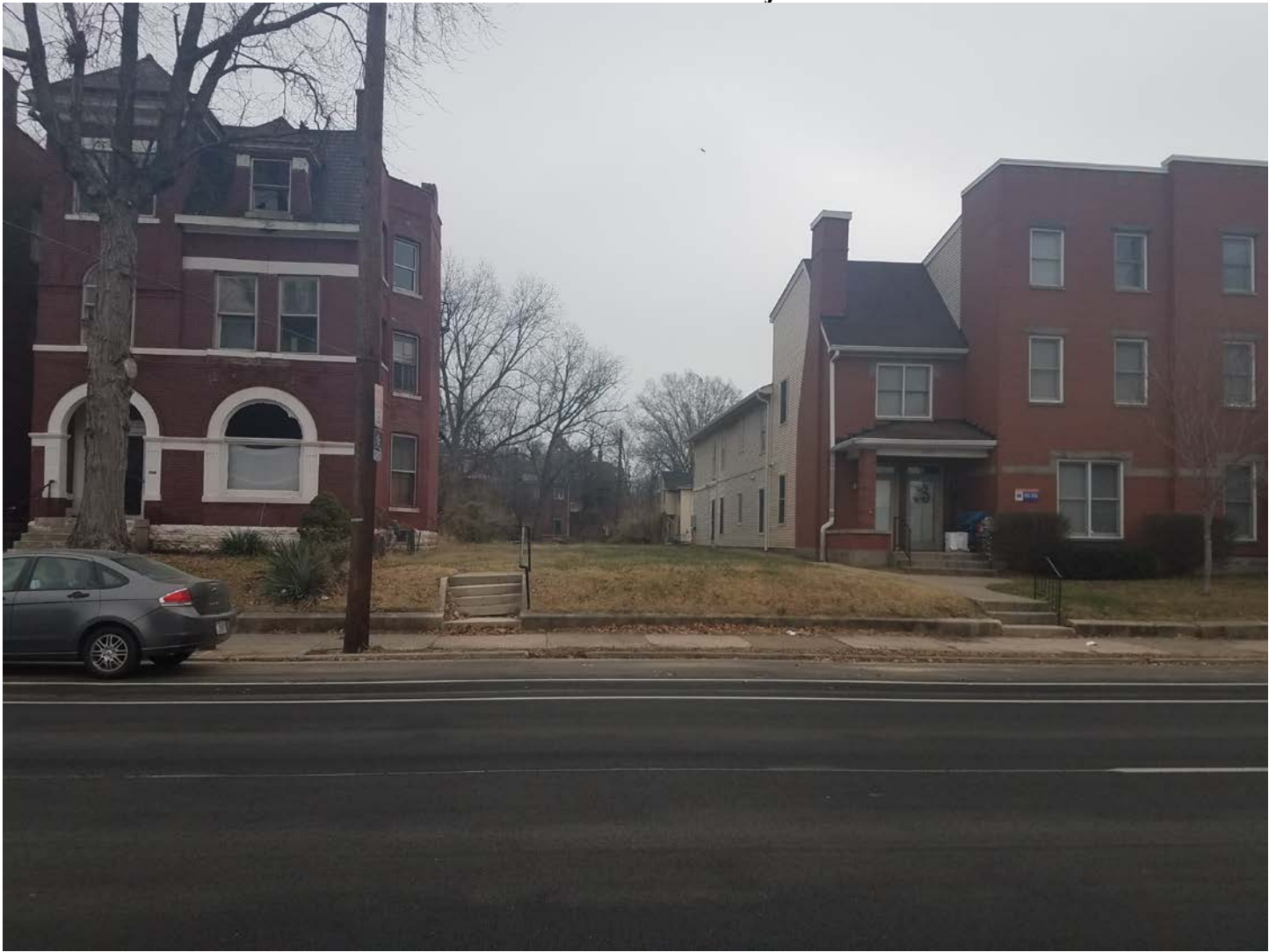
Photo 1: 1133 S. 2nd Street - Subject Photo
