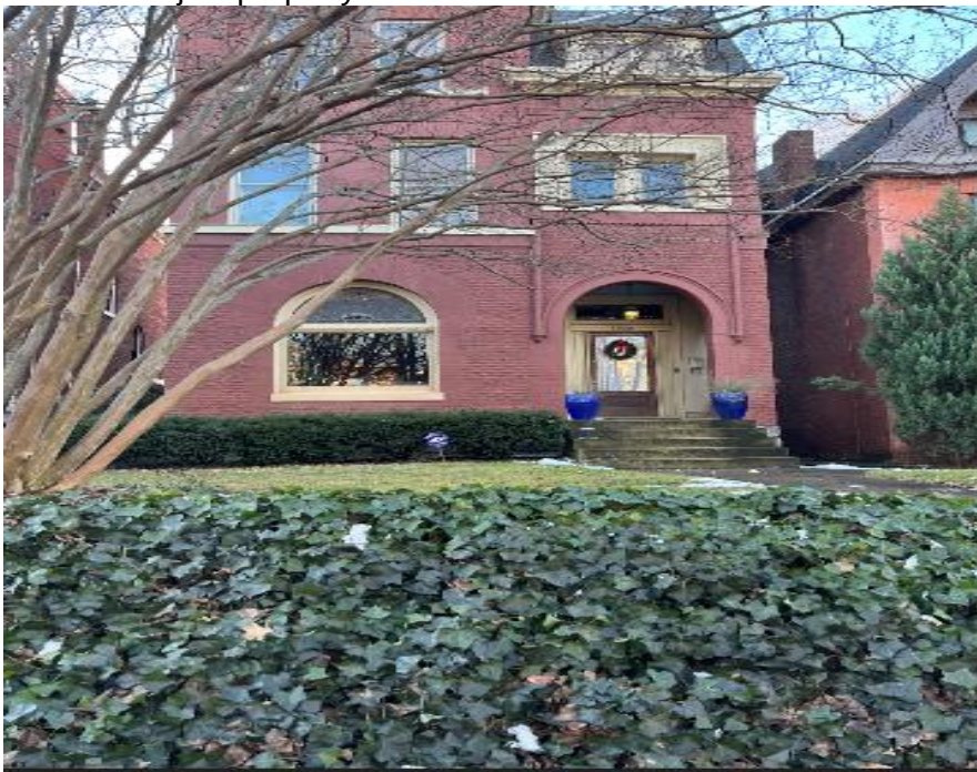
Right of the subject property.
