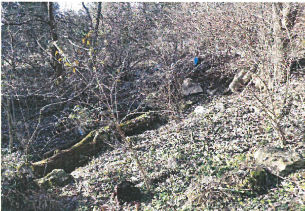
Area 01a – minor erosion
