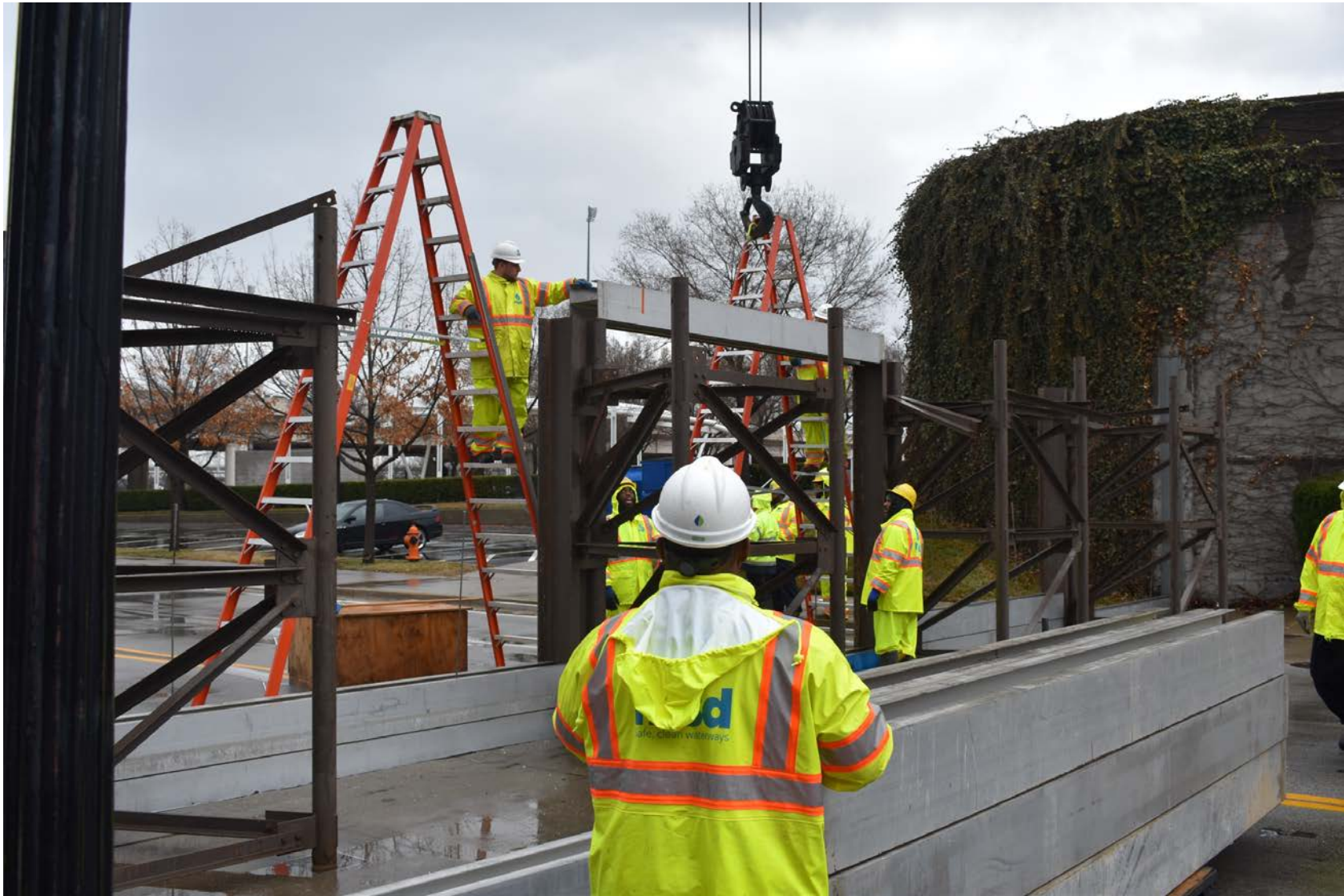
Bingham Way Street Closure
