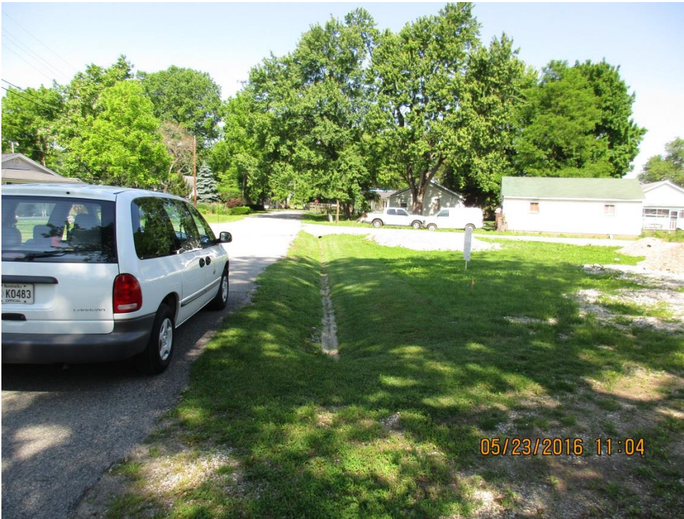
Looking along the subject site frontage along Albany Ave., the applicant is requesting a waiver from having to provide a sidewalk. (Sidewalk waiver and waiver #3)
