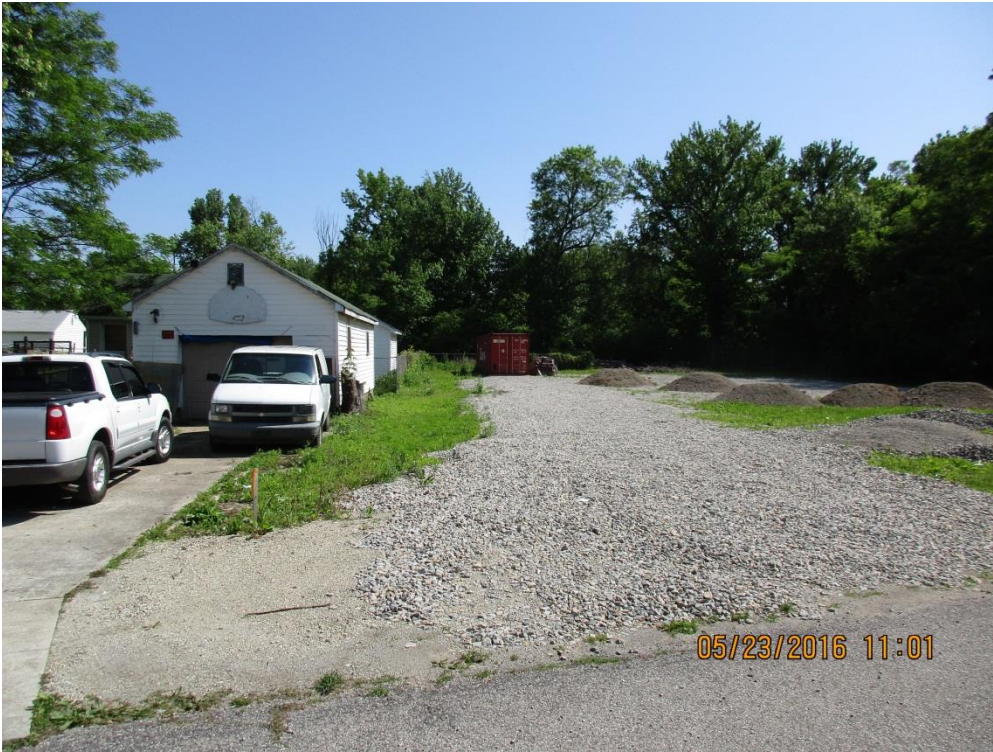
Looking along the western property where a 6 foot continuous screen would be required. Applicant is requesting a waiver (variance and waiver #5).
