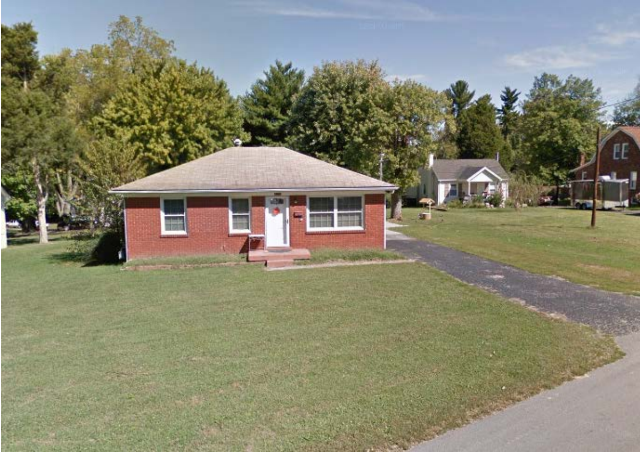
The property to the right of the subject property.
