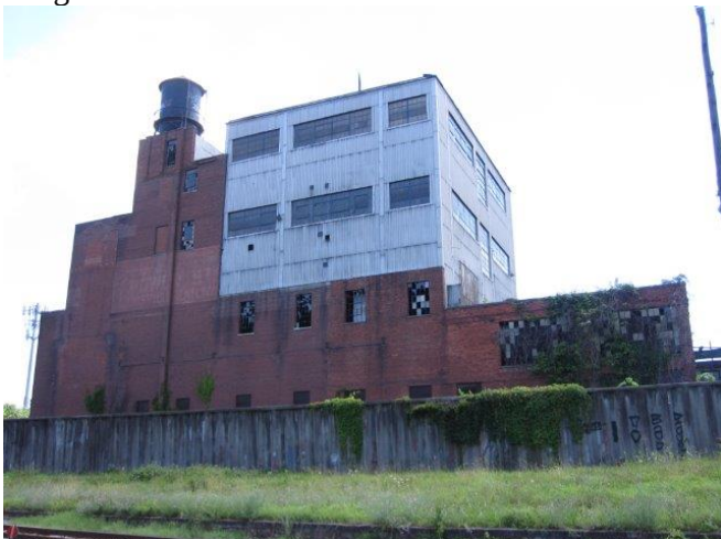
Northeast façade (river side). Floodwall in foreground
