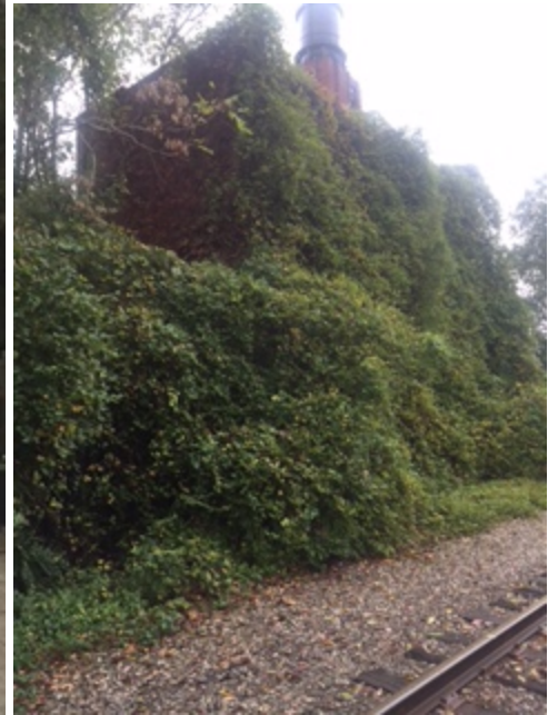
Screenhouse from tracks, looking west
