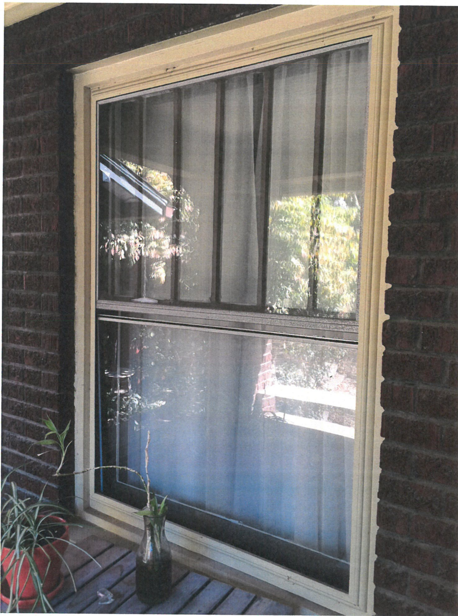
Front Façade Window #4 left of the door.
