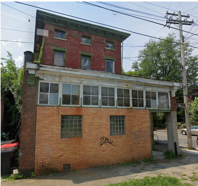
Google Streetview, June 2021, showing damage
