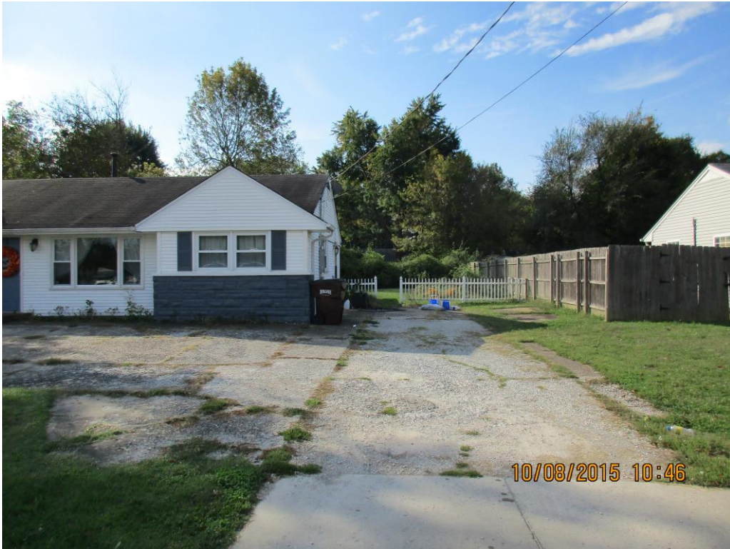
Front of the existing house
