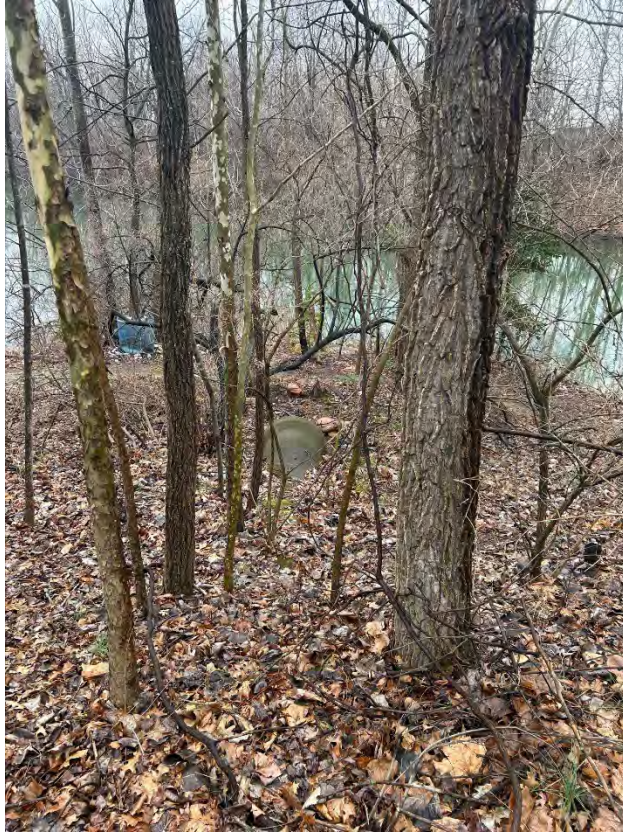
Northeastern Storm Sewer Outlet
