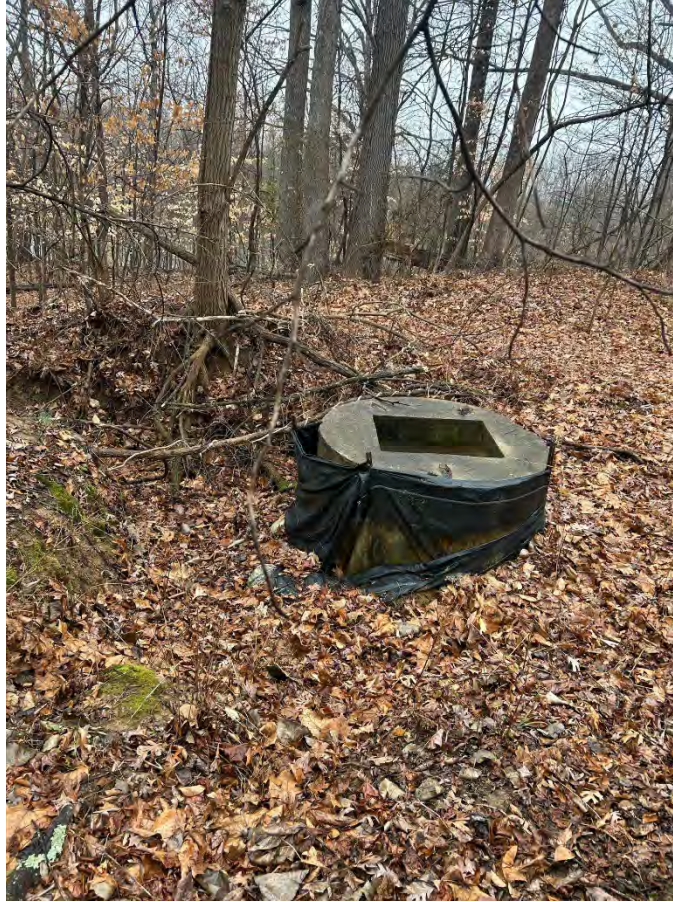
Southern Storm Sewer
