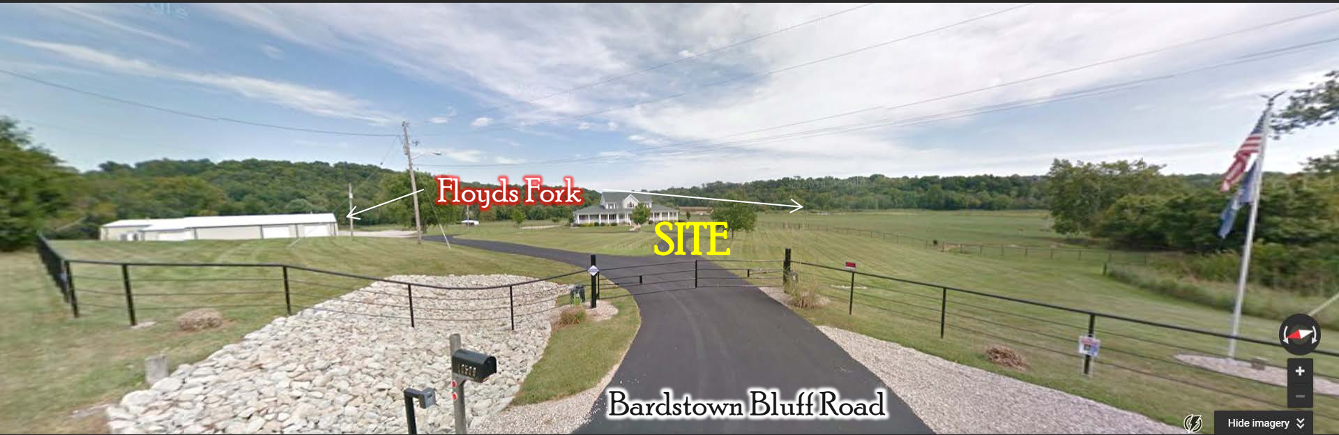
View of site from Bardstown Bluff Road
