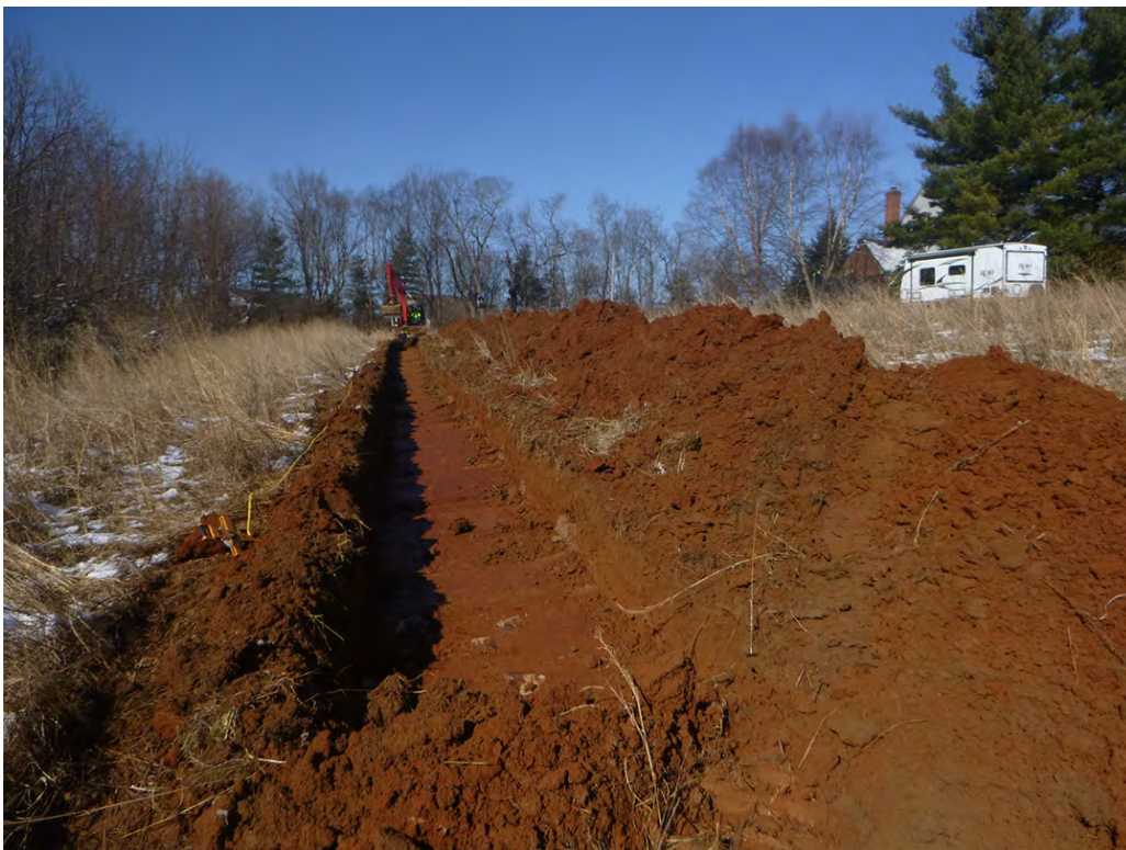
Figure 12. Photograph of Trench 3 Looking North.
