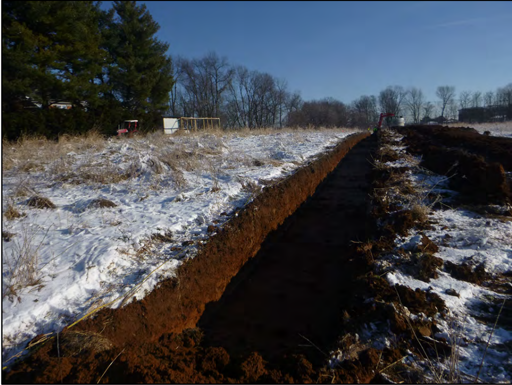
Figure 11. Photograph of Trench 1 Looking Northeast.
