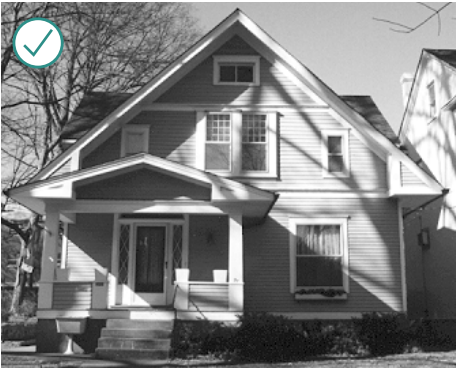
Preserve an original porch in its original location. An original porch enhances the design of a single facade and unifies an area of a preservation district through repetition of form.
