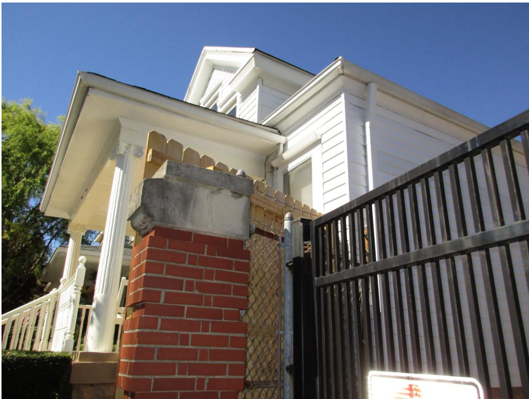
Existing 7-8' security barbed wire fence
