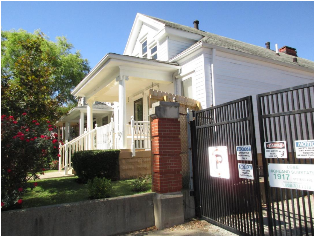
Existing 7-8' security barbed wire fence
