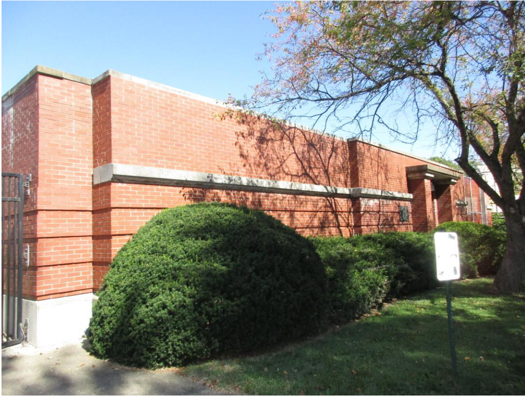
Existing brick wall around a portion of the LG&E substation
