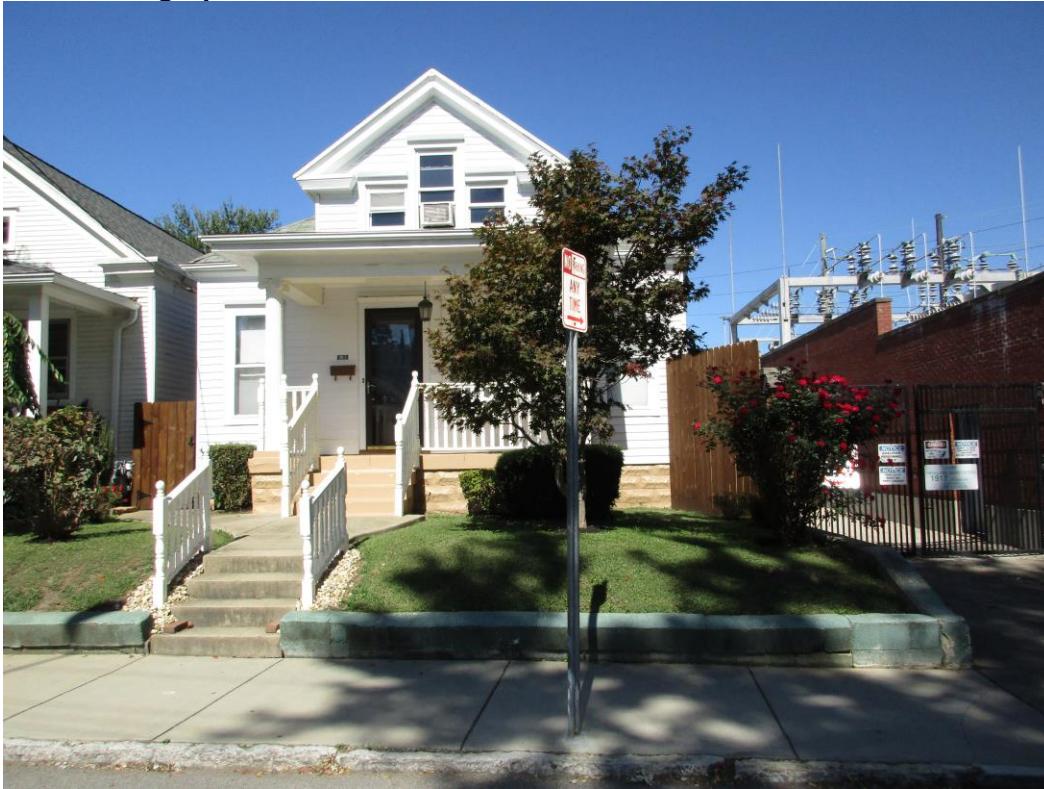
Front of the home
