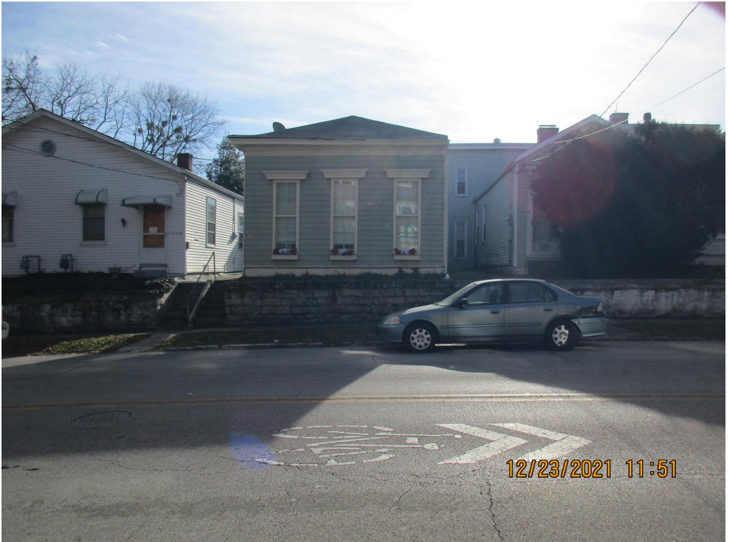
Front of subject property.
