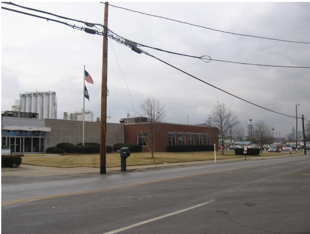
Existing sidewalk along Zeon property on south side of Bells Lane
