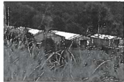
JEFFERSON COUNTY PROPERTY VALUATION ADMINISTRATOR An event venue that could host weddings, Derby parties and other events has been proposed on this site in existing horse barns next to the Parklands of Floyds Fork.
