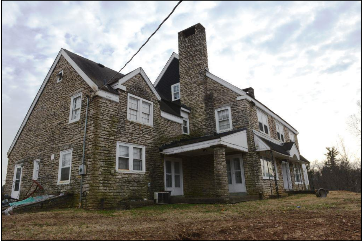
Image 7. Northeast elevation of 609 Blankenbaker Lane.
