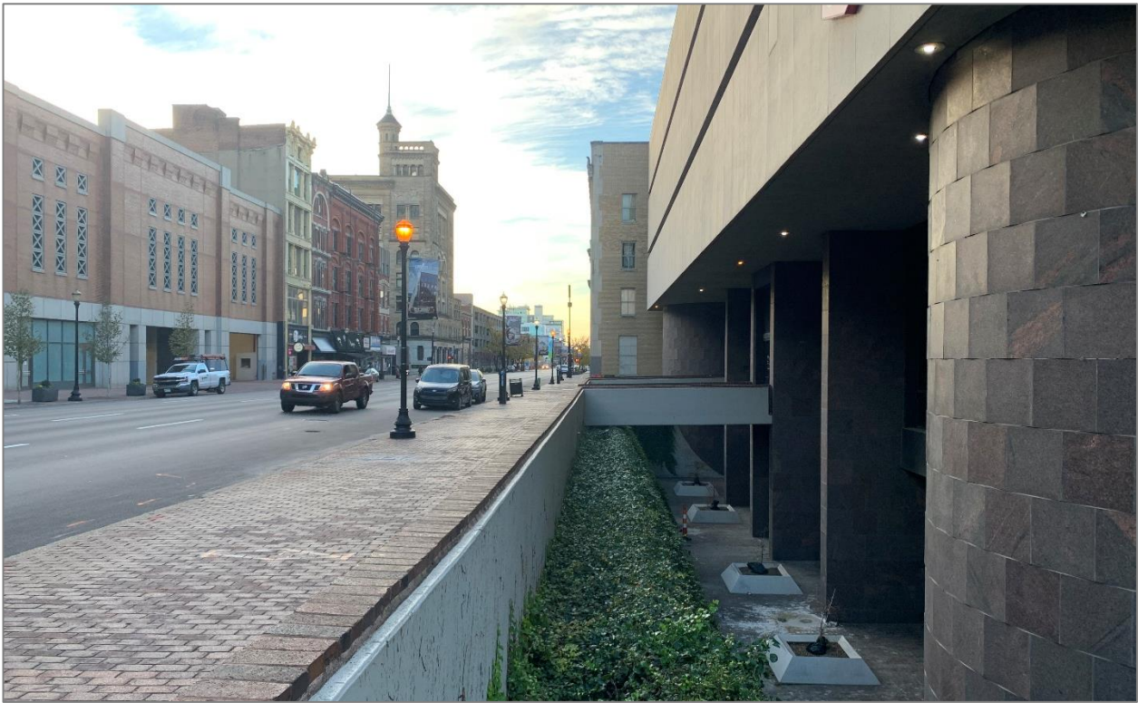
W Market Entrance and Lower Plaza November 30, 2021
