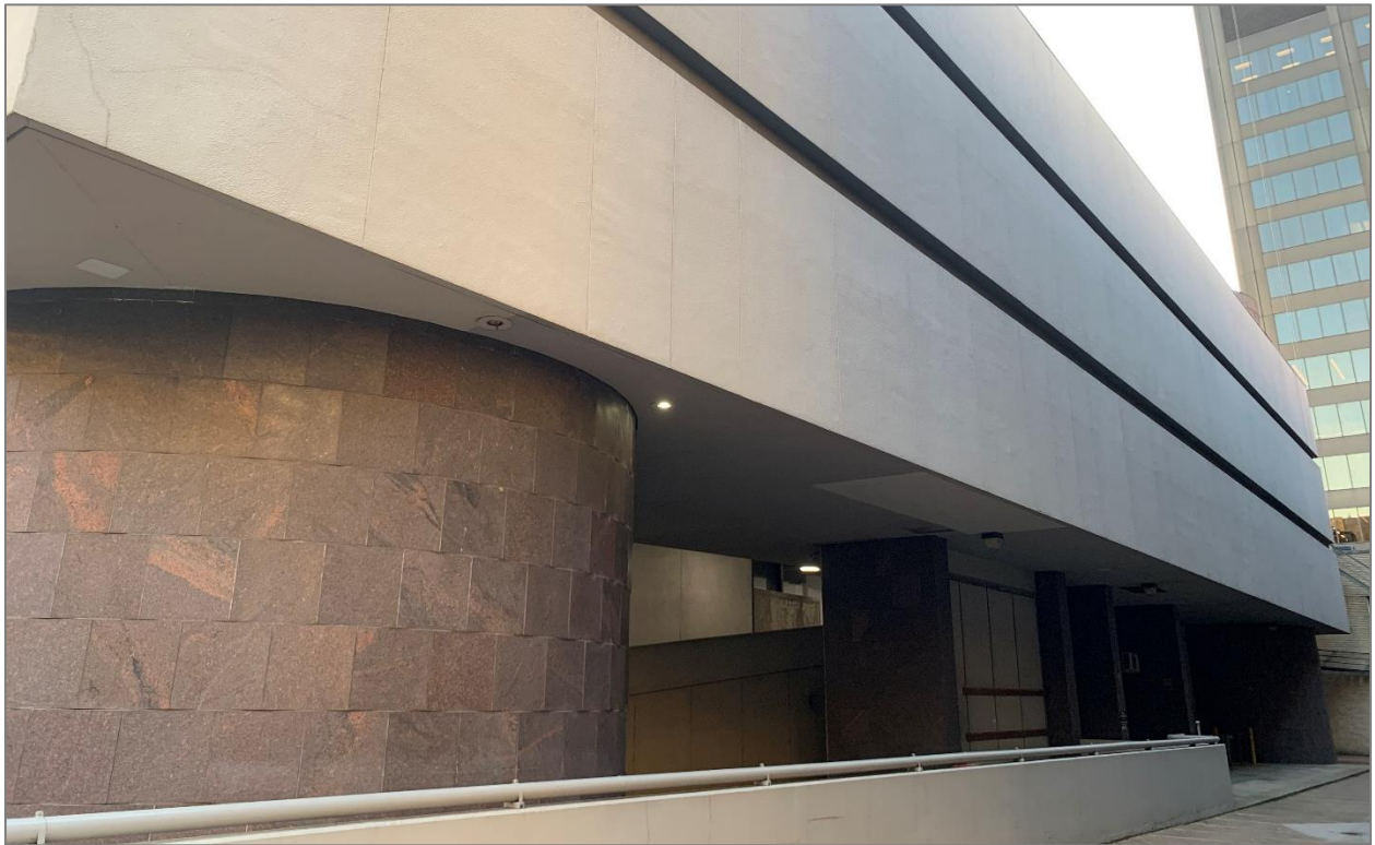
Northern Building Façade November 30, 2021
