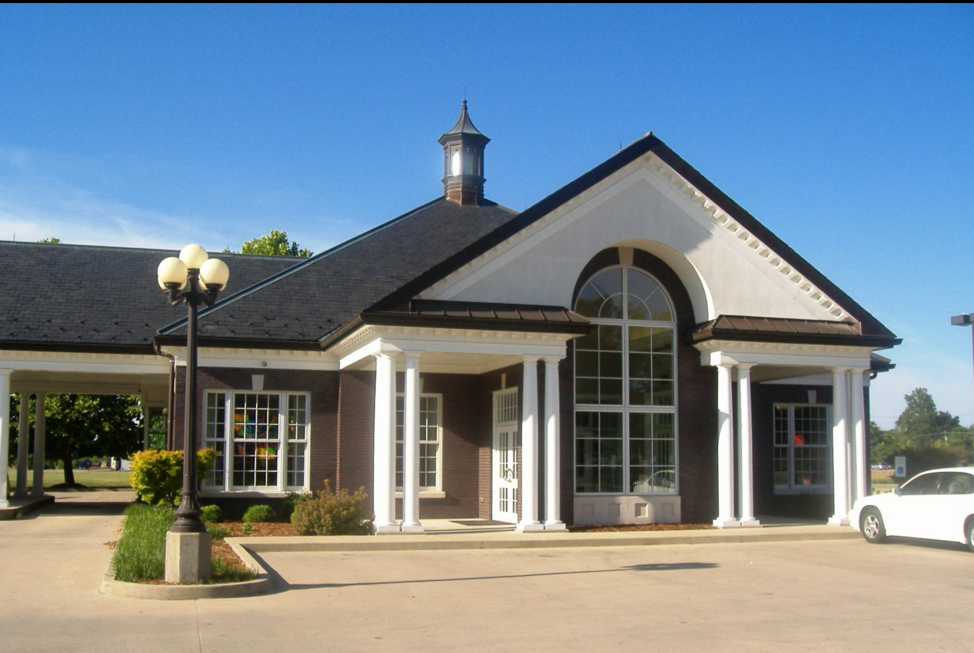
Branch bank on Greenwood Road in Pleasure Ridge Park
