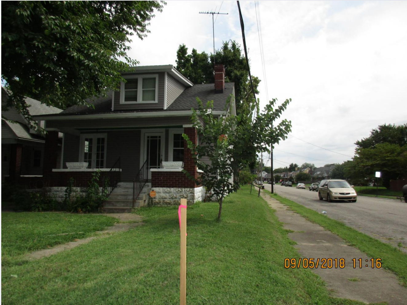
Looking down the street side yard.
