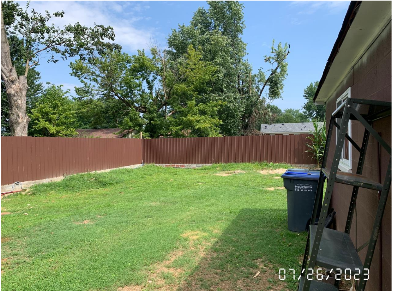
Fence in the rear yard.
