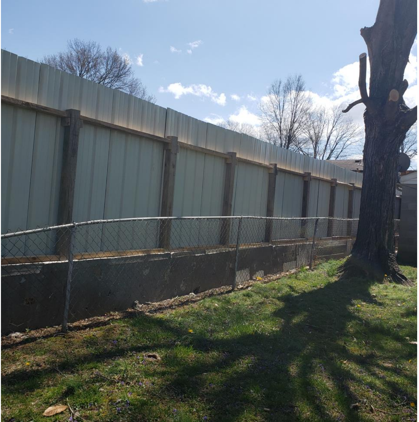
Backside of fence on rear property line.
