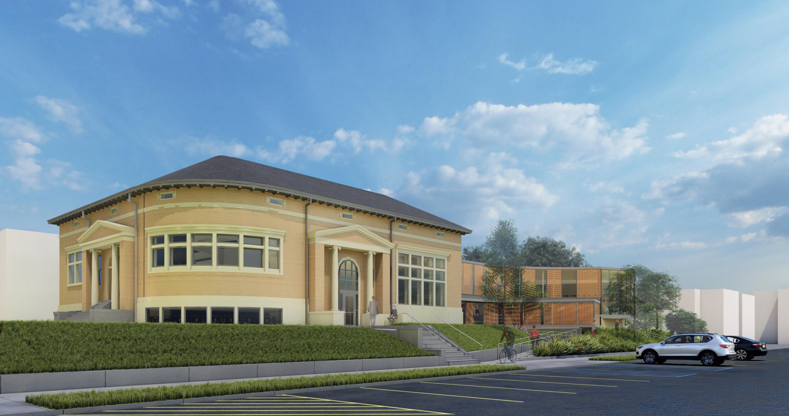
EXTERIOR VIEW FROM NORTHWESTERN PARKWAY & 33 RD
