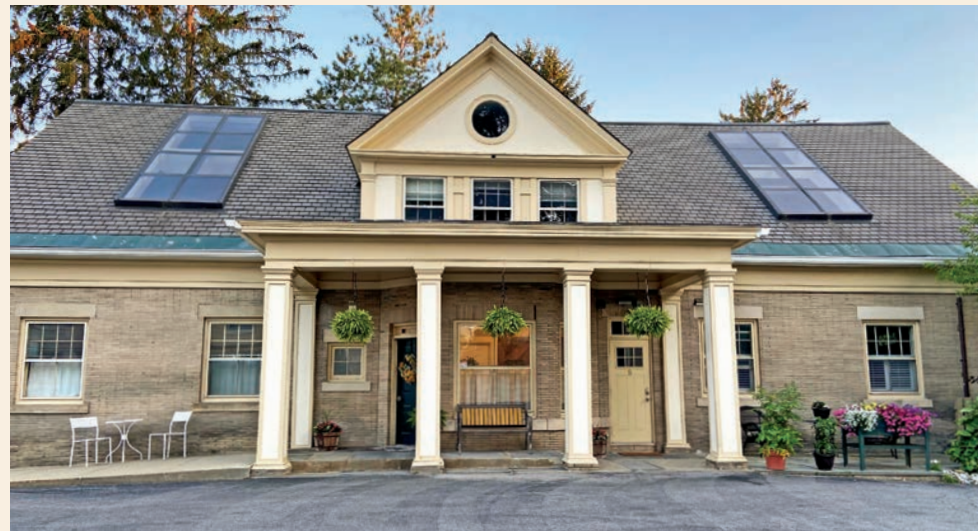
◀ Few older homes meet accepted accessibility standards. In fact, historic examples of Missing Middle Housing frequently feature a raised first floor. This 5,000-square-foot building in Saratoga Springs, New York, with a zero-step entrance is an exception. Built in 1930 as office space for Skidmore College, the property is now a five-unit residence with three apartments downstairs and two up top, including two studios, two one-bedroom units and one two-bedroom unit.
