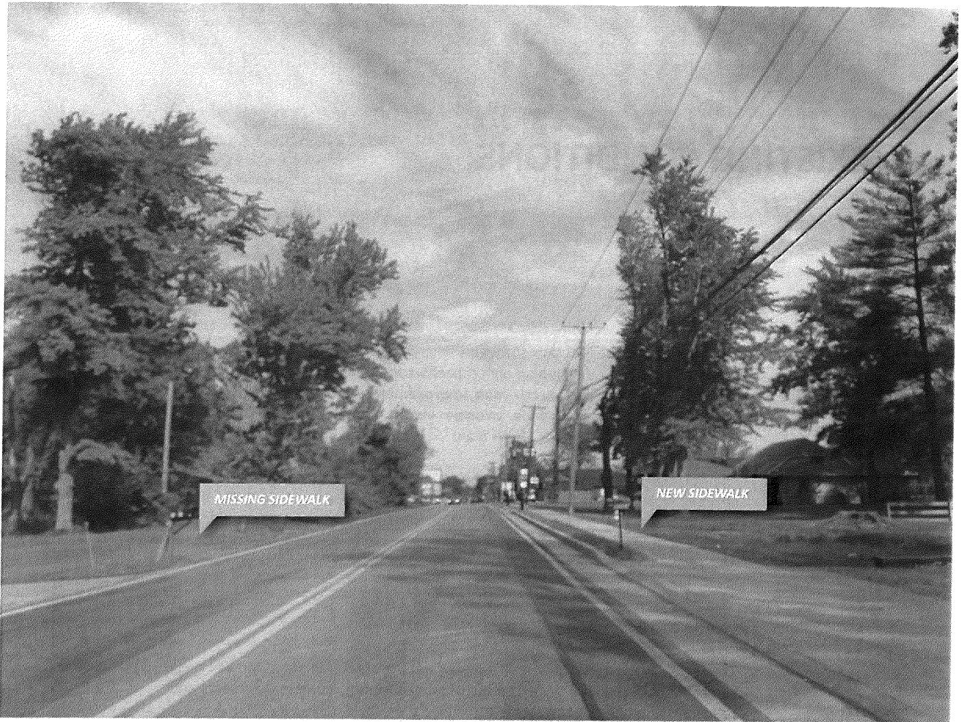
Figure 2.15 - Missing Sidewalk on Fegenbush Lane
