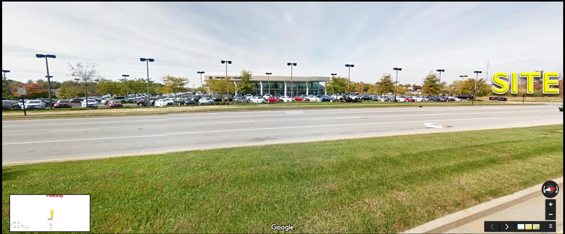
View of existing Lexus dealership along Blankenbaker Parkway. Site is to the right (north) of the Lexus dealership.
