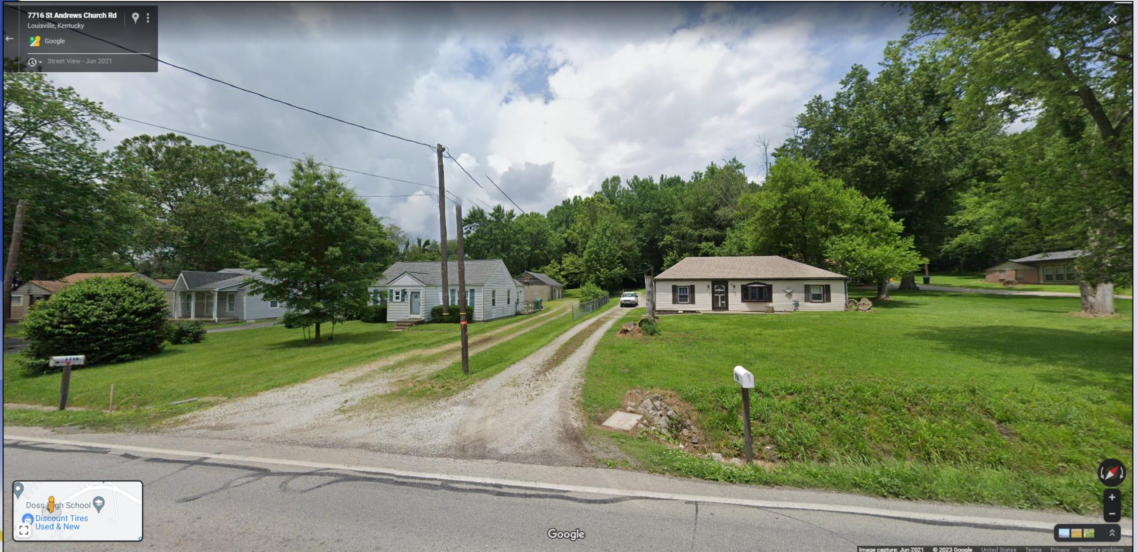
Residential across St Andrews Church Road
