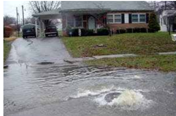
Sewer manhole overflow in Louisville. Image Source: MSD Project Win
