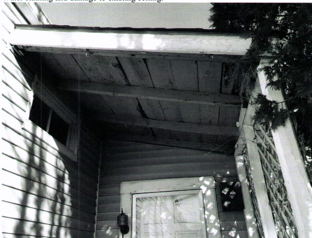
Side door porch roof framing.
