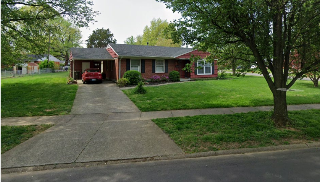
Front of subject property (Google Street View)
