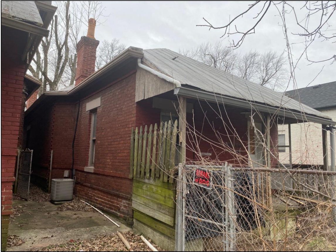
Figure 11. Rear (north) elevation, looking southwest.
