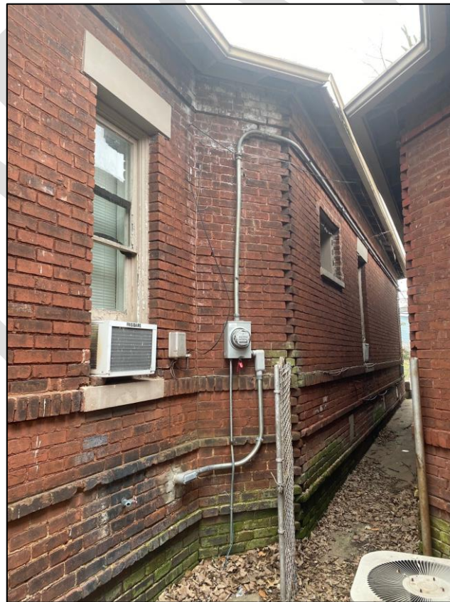
Figure 15. West elevation, looking south.
