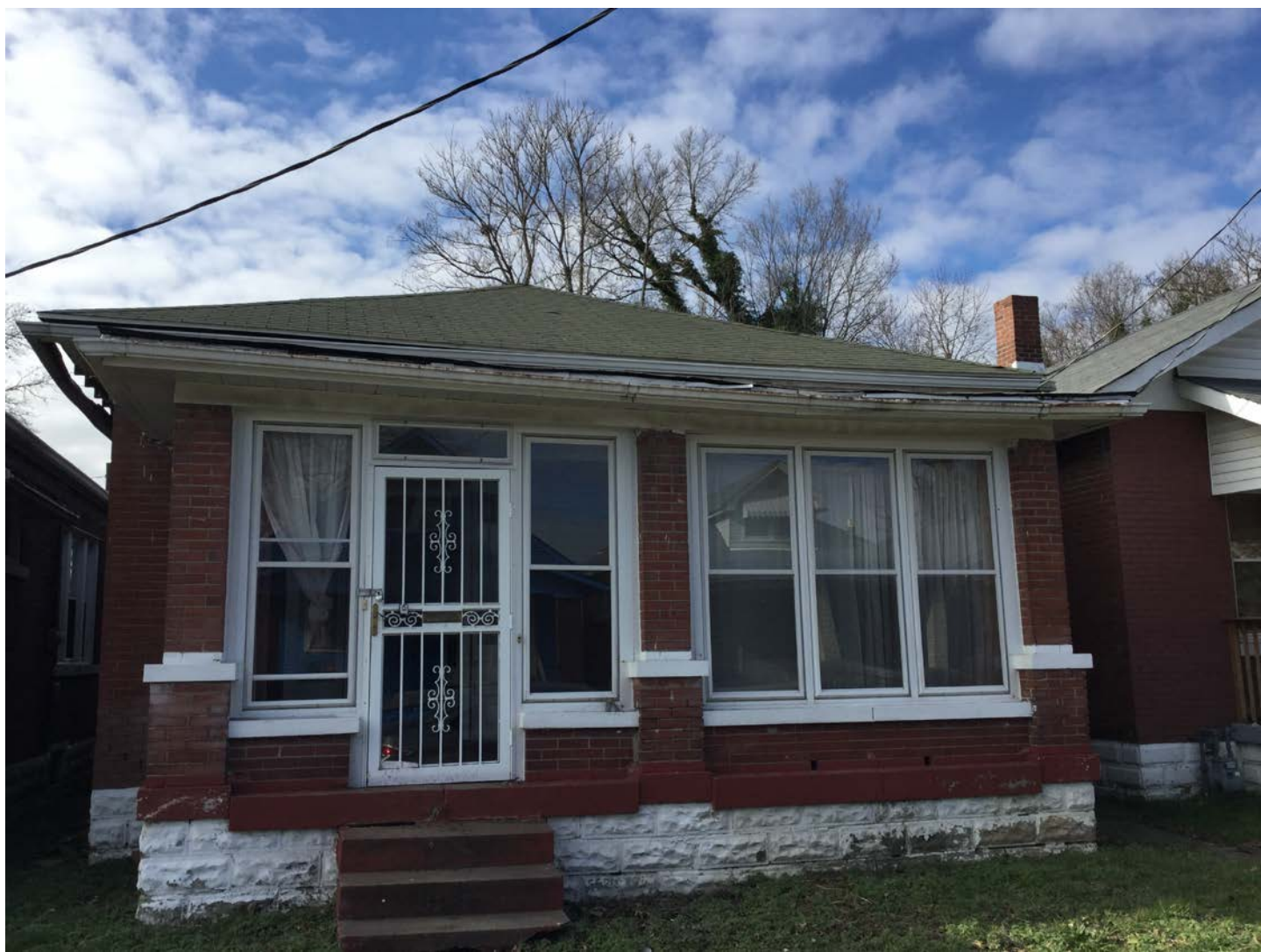
726 Sutcliffe Ave Front View
