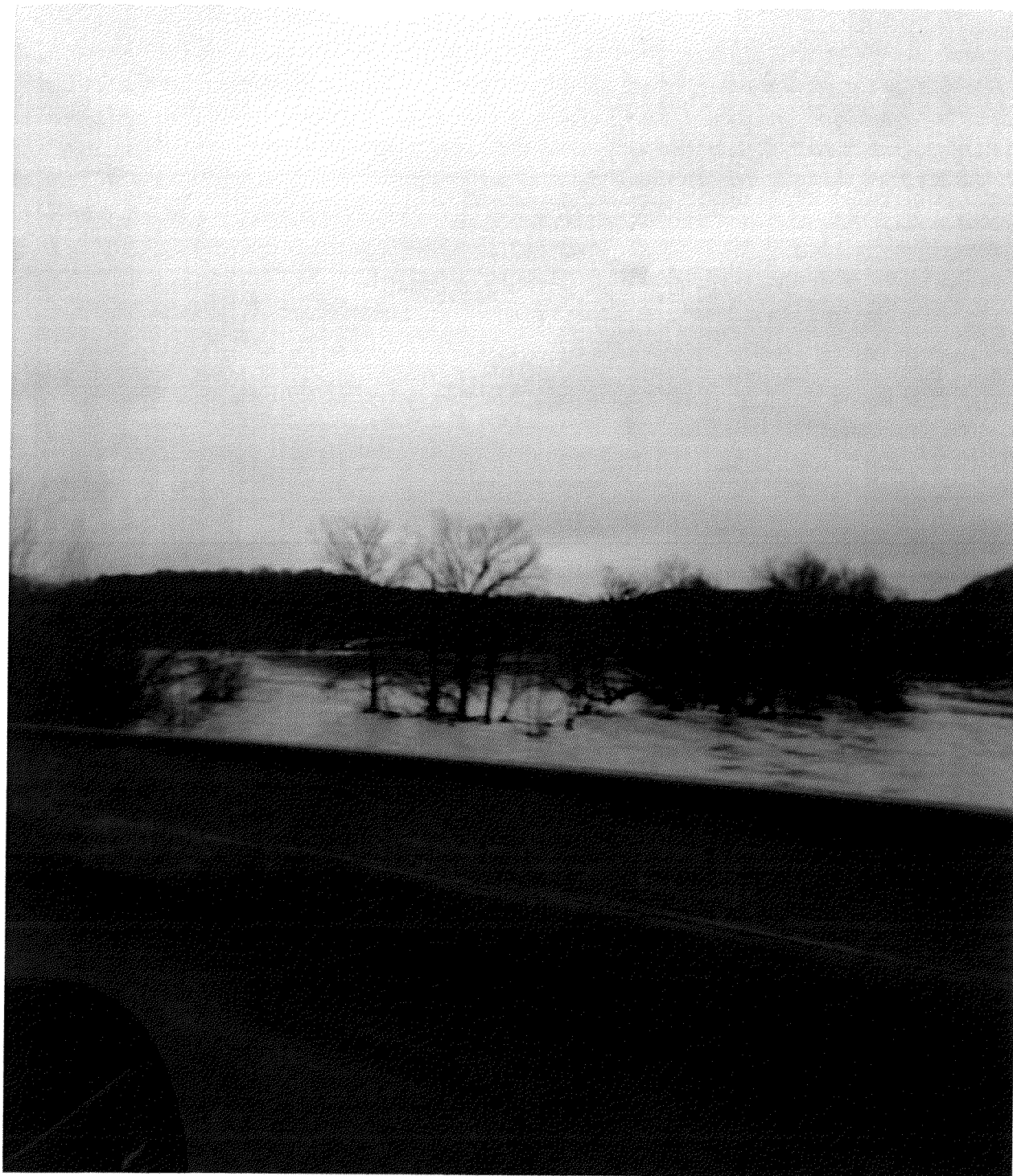
Bardstown Road Bridge with water dangerously close to the top of the bridge. In the back ground is the Floyds Fork park bridge.
