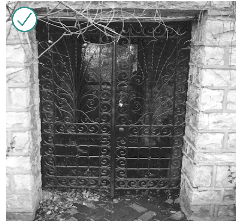
Install security bars of simple design that do not obscure the architectural character of the original doors or damage historic fabric. Here, a historic metalwork door secures an Old Louisville entrance.
